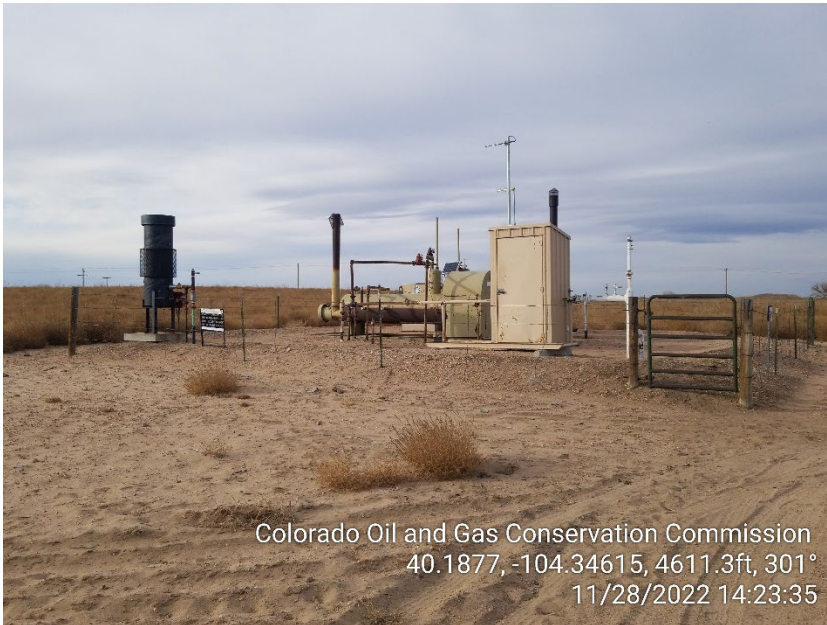
Photo 5 – Separators, ECD and Gas Meter
