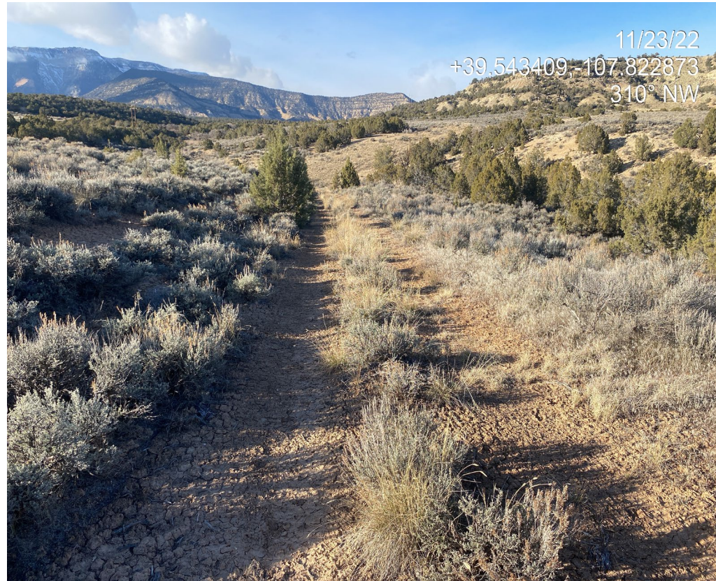
Photo 2. Photo shows the access road remains. Portions of the two-track to the south of the culvert lack vegetation in tracks and require additional reclamation. Note center of road is well vegetated.
