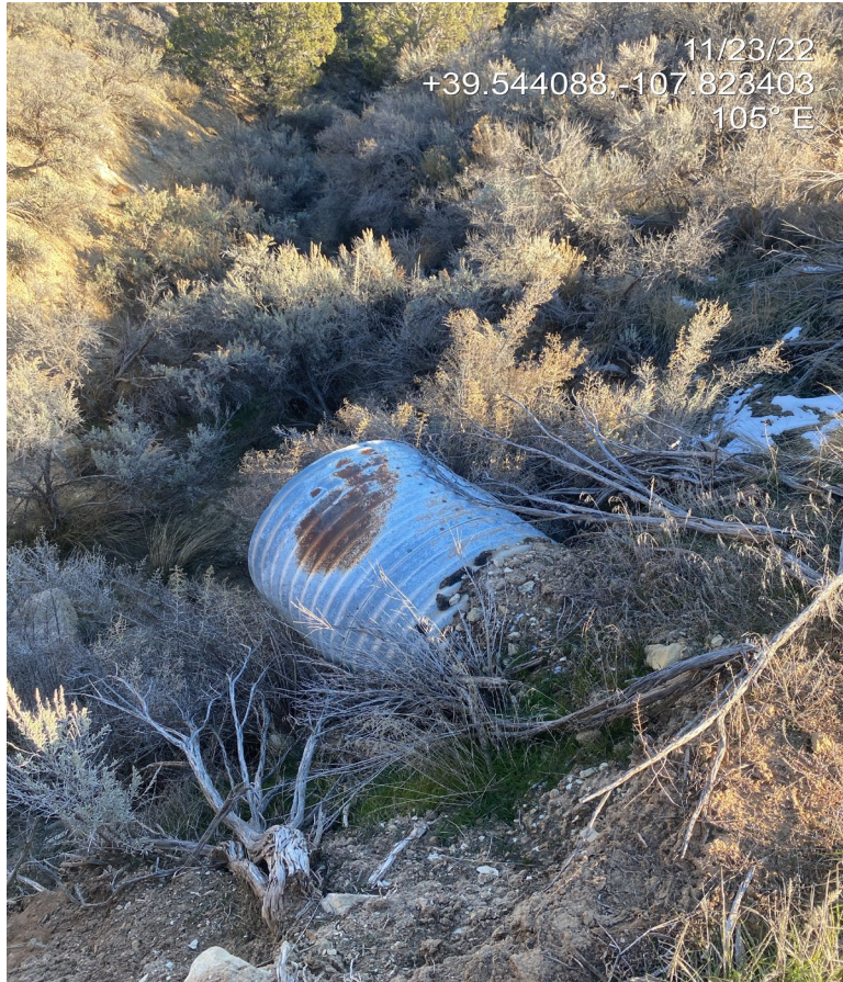
Photo 1. Photo shows the access road culvert remains.
