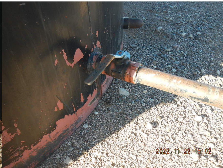
Photo 6. Oil weeping from valve and fittings.
