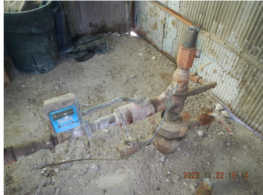
Photo 14. Oil staining around valve threads and on the ground.
