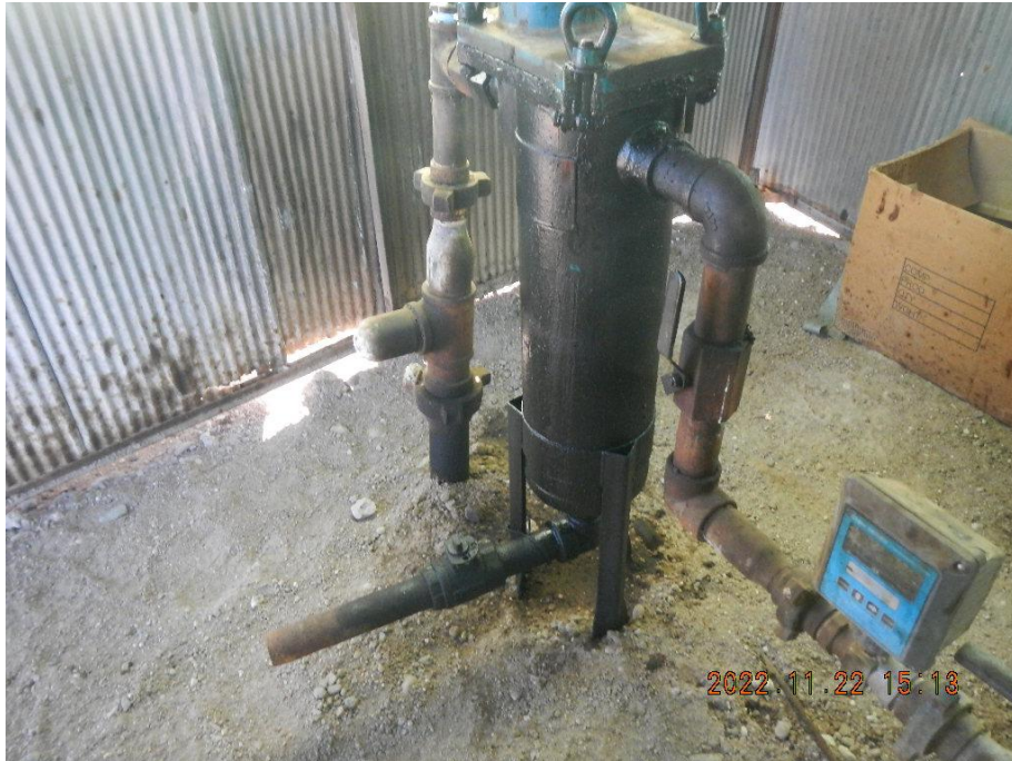
Photo 13. Filter with oil staining and oil staining on the ground.
