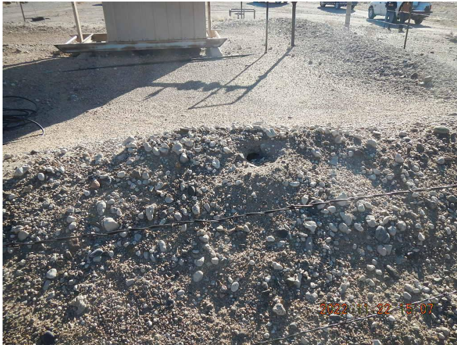
Photo 9. Burrows compromising secondary containment berm.
