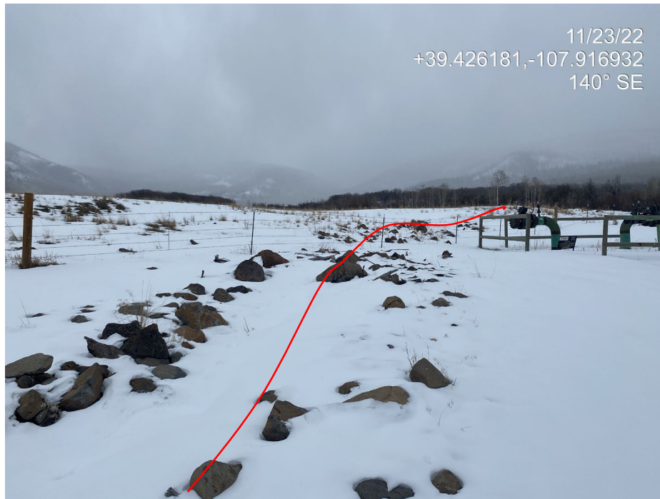
Photo 3. Photo taken from the western edge of the location shows a stormwater ditch which must be removed for the location to pass final reclamation. Line indicates where the ditch continues onto the location.
