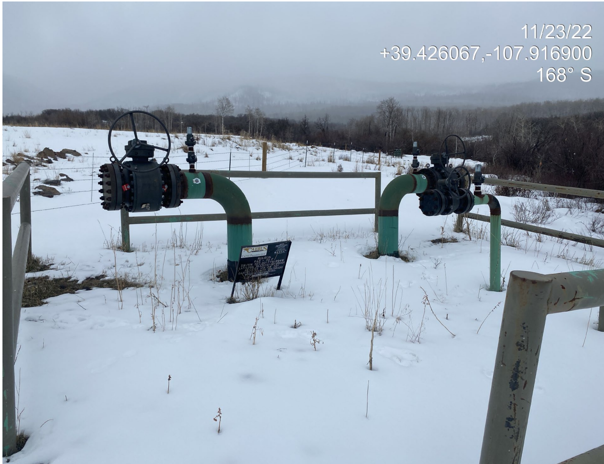
Photo 5. Photo shows three (3) risers at the northwest of the location. Risers must be removed per 1004 Rules.
