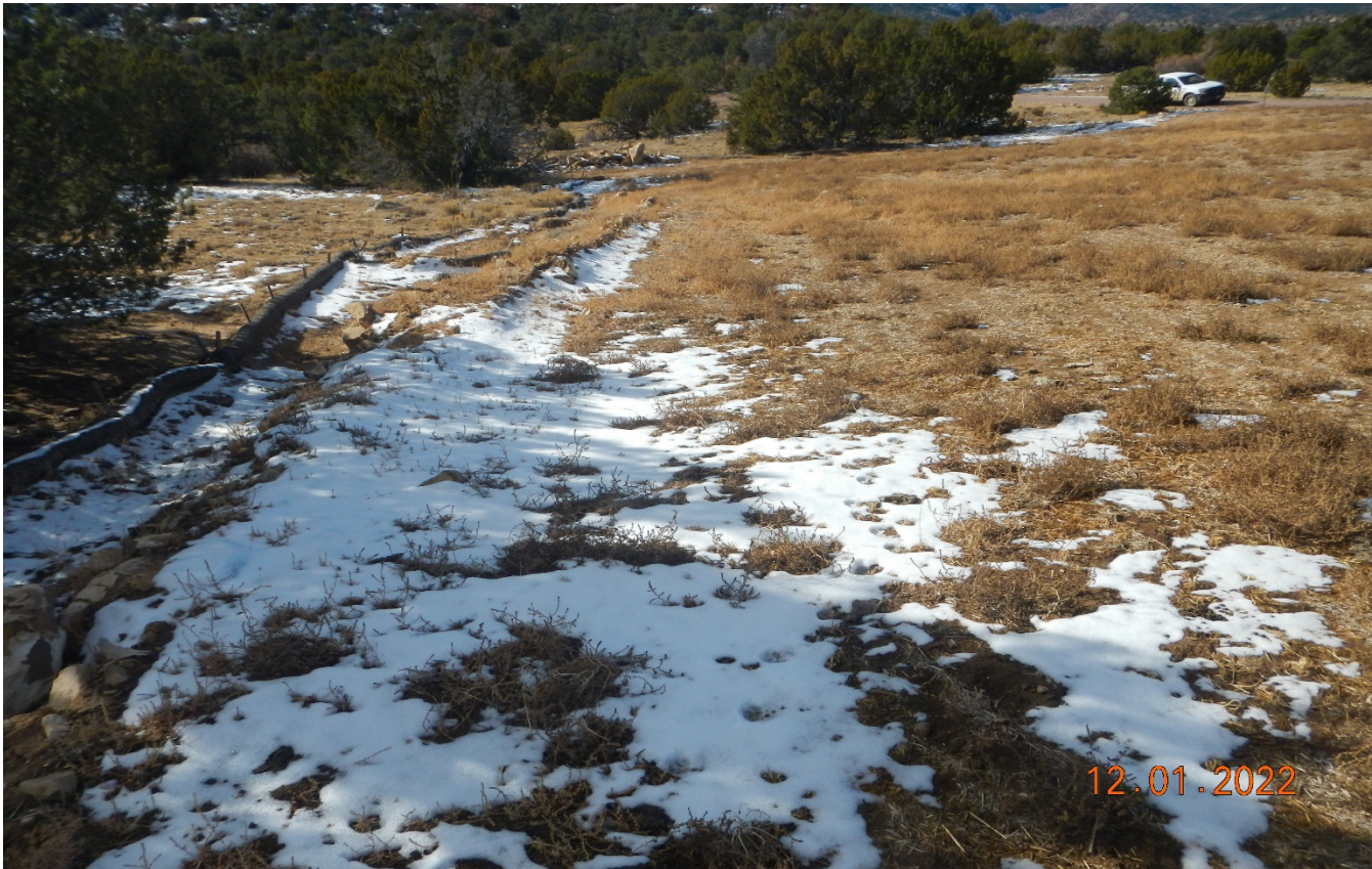
Photo 7. Facing south at the east side of the location. There are some wattles in this area that are displaced and need maintenance.
