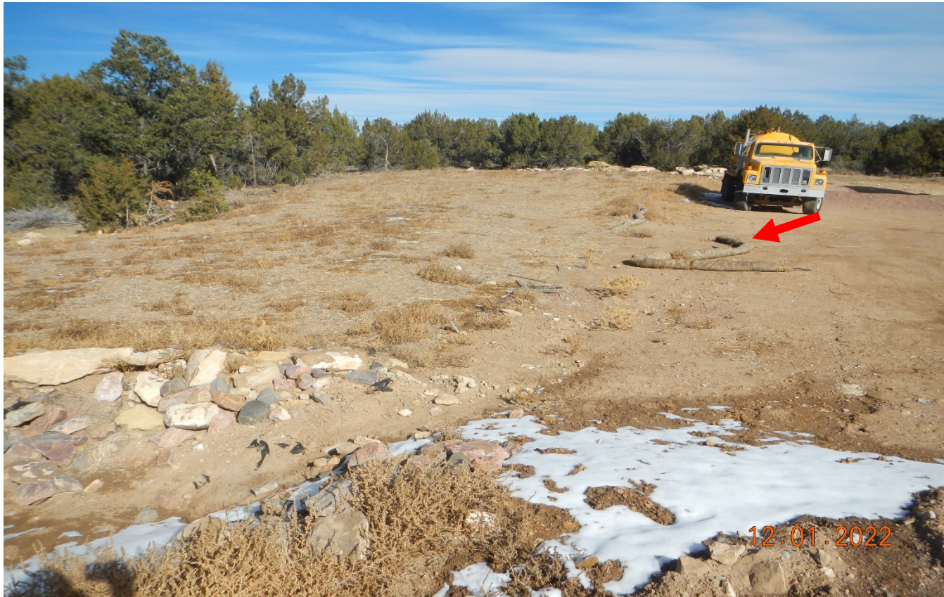
Photo 4. The topsoil pile has mostly been used for interim reclamation. This area appears to have been seeded and mulched but vegetation has not yet established. There are displaced wattles that need to be reinstalled.
