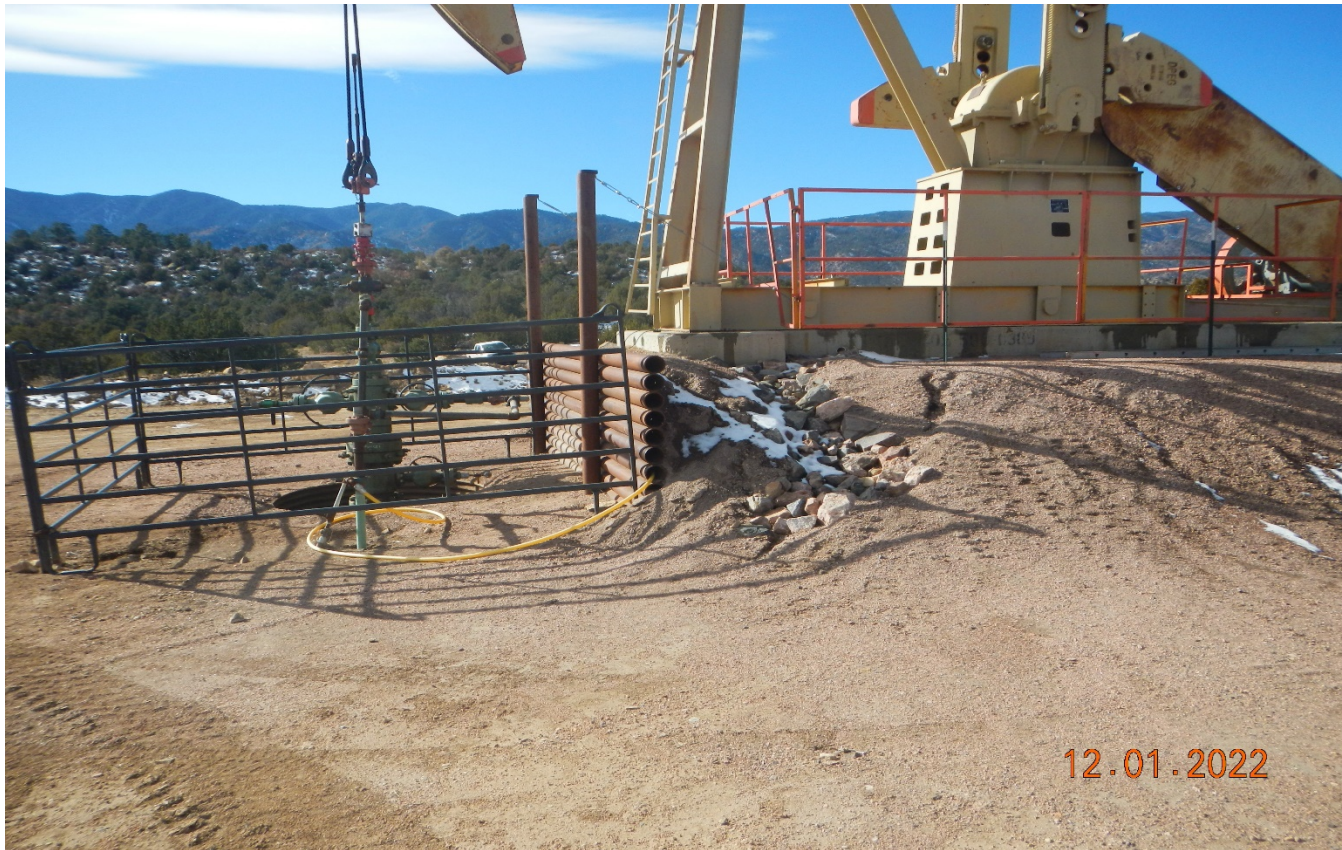
Photo 6. Facing toward the pumpjack. Erosion was repaired with rock ri/rap.
