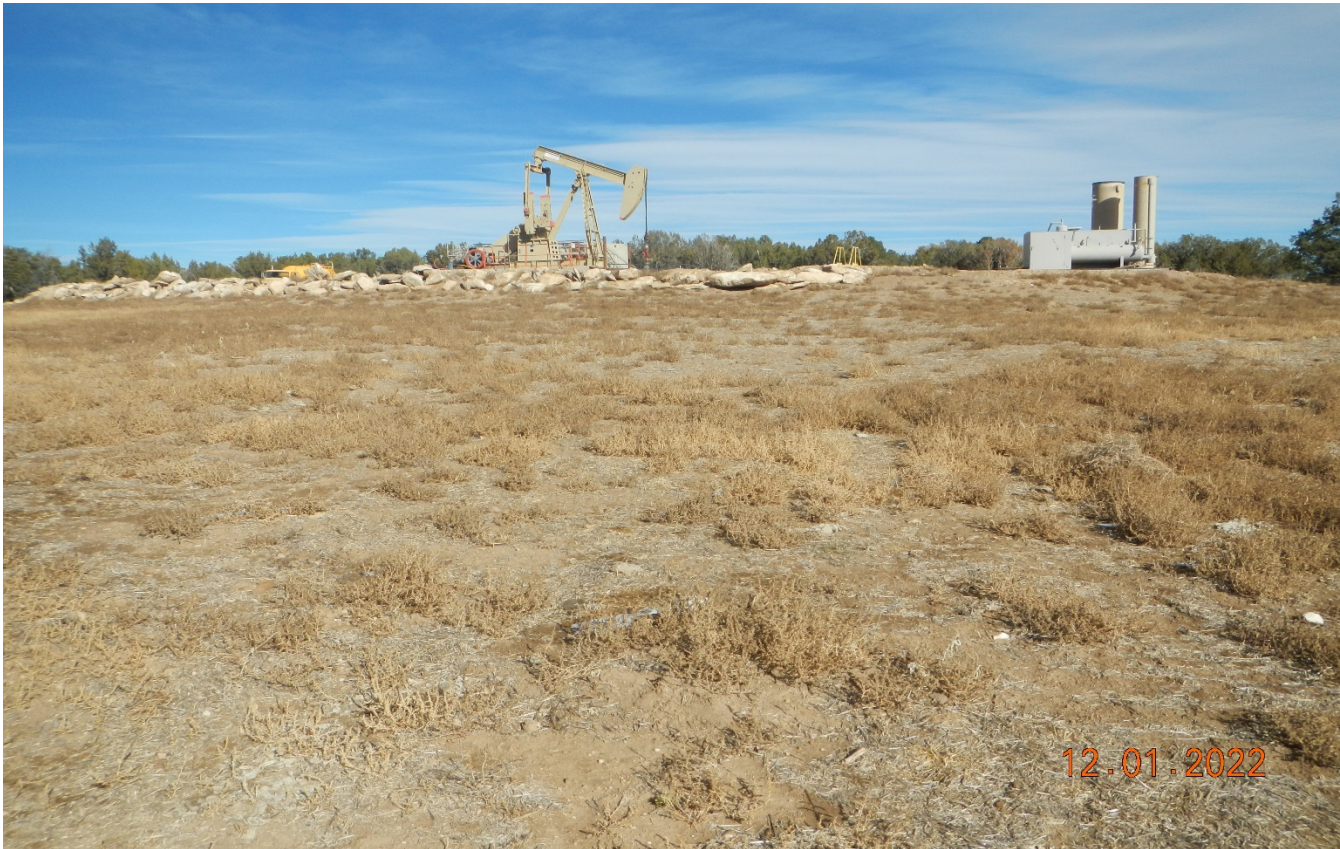
Photo 8. Facing northwest toward the location. The interim reclamation area appears to have been seeded and mulched but vegetation has not yet established. There are mostly undesirable weeds which will need to be controlled.
