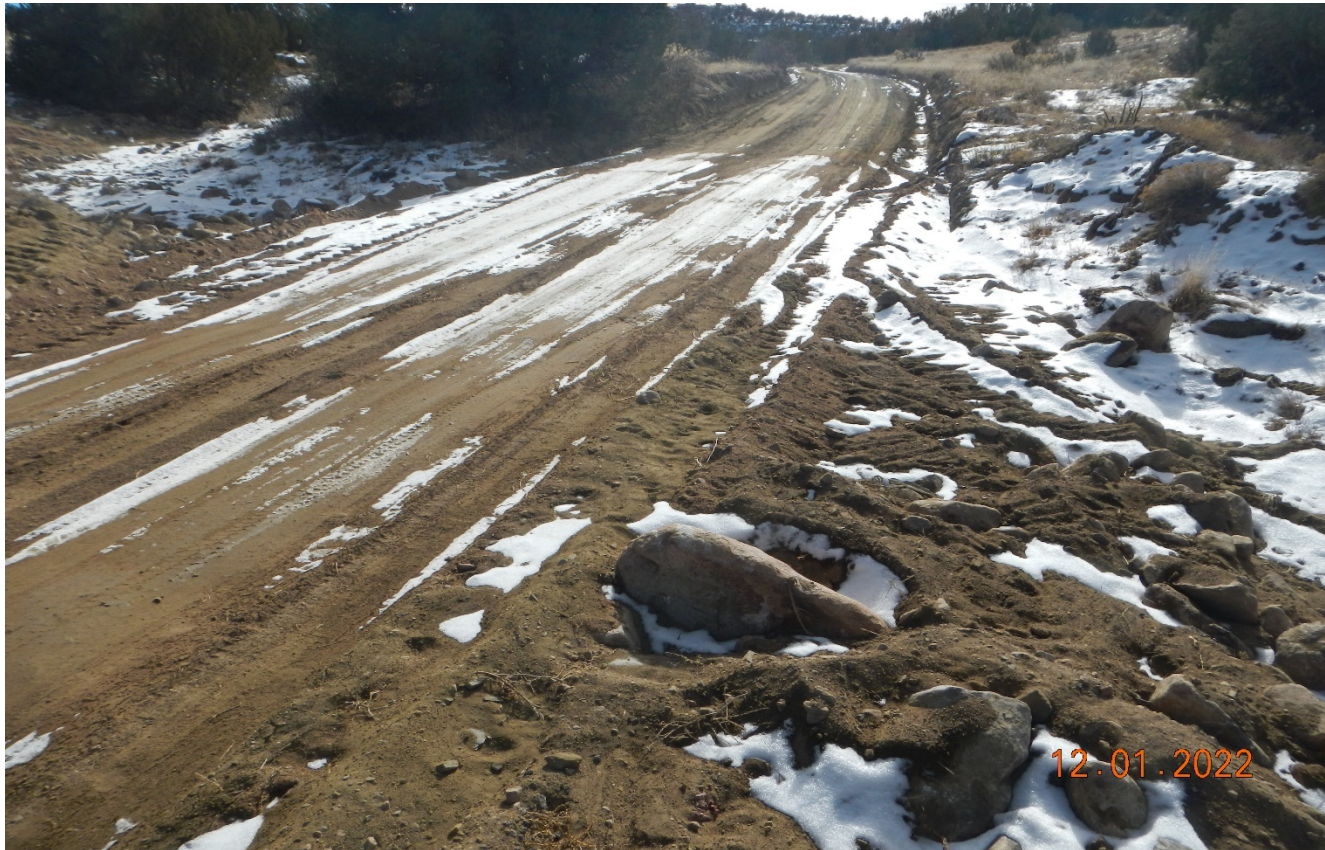
Photo 1. Facing southeast long the access road. This drainage crossing must have BMP's installed to accommodate seasonal storm event to prevent material from washing out. BMP may include culvert, rip/rap, ect.
