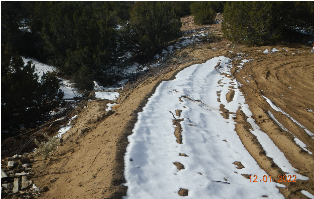
Photo 5. The soils have been pushed out and disturbed and are susceptible to erosion. Disturbed soils need to be stabilized.
