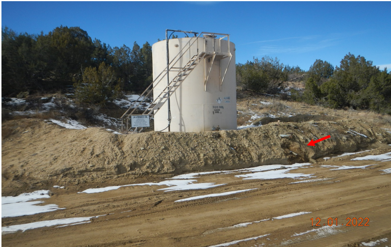
Photo 2. Facing toward the tank battery. There is still stained soils at the berm.
