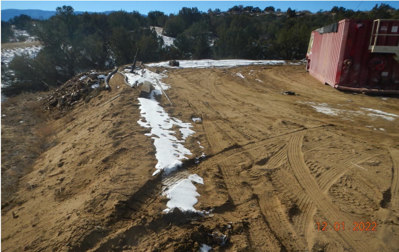
Photo 4. Facing southeast along the fill slope of the pad. The soils have been pushed out and disturbed and are susceptible to erosion. Disturbed soils need to be stabilized.
