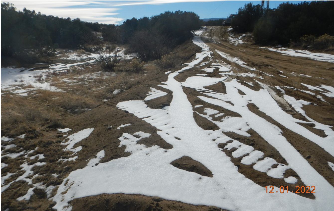
Photo 3. Facing southeast along the access road. The soils have been pushed out and disturbed and are susceptible to erosion.
