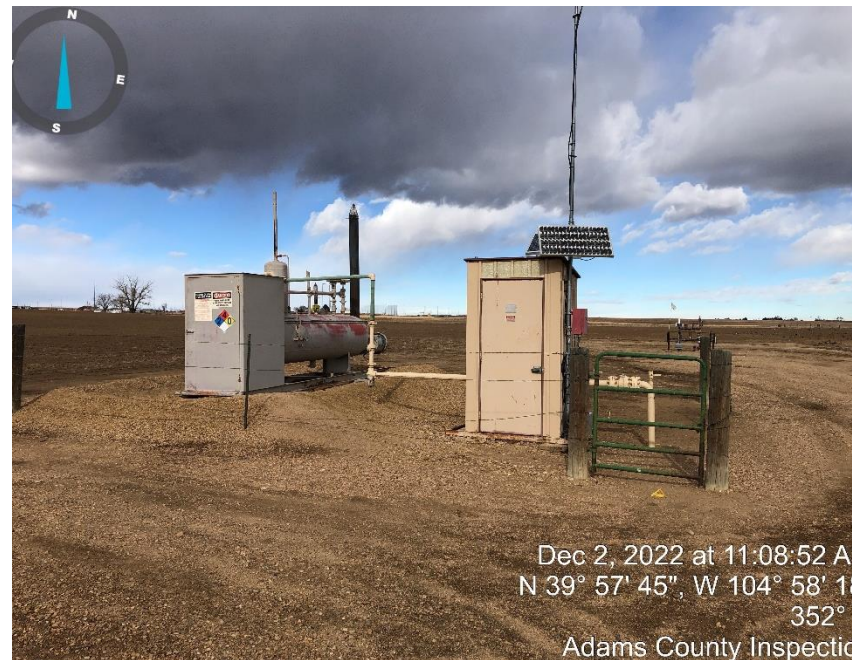
Photo# 2 Separator & Meter house.
