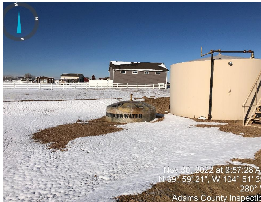
Photo# 2 P/W tank.
