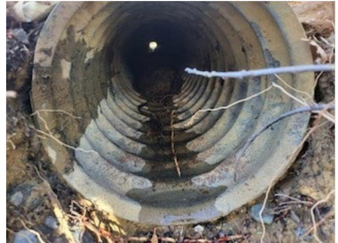
Sediment removed and drainage ditch established on back side of location
