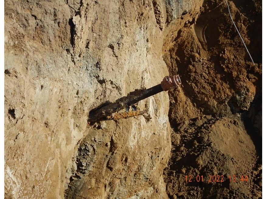
Flowlines exposed in excavation prior to completion of repair; (1) 2" CS OLF (cut end ball valved); (1) 1" CS OOS (historical gas supply) flowline (cut end not sealed).
