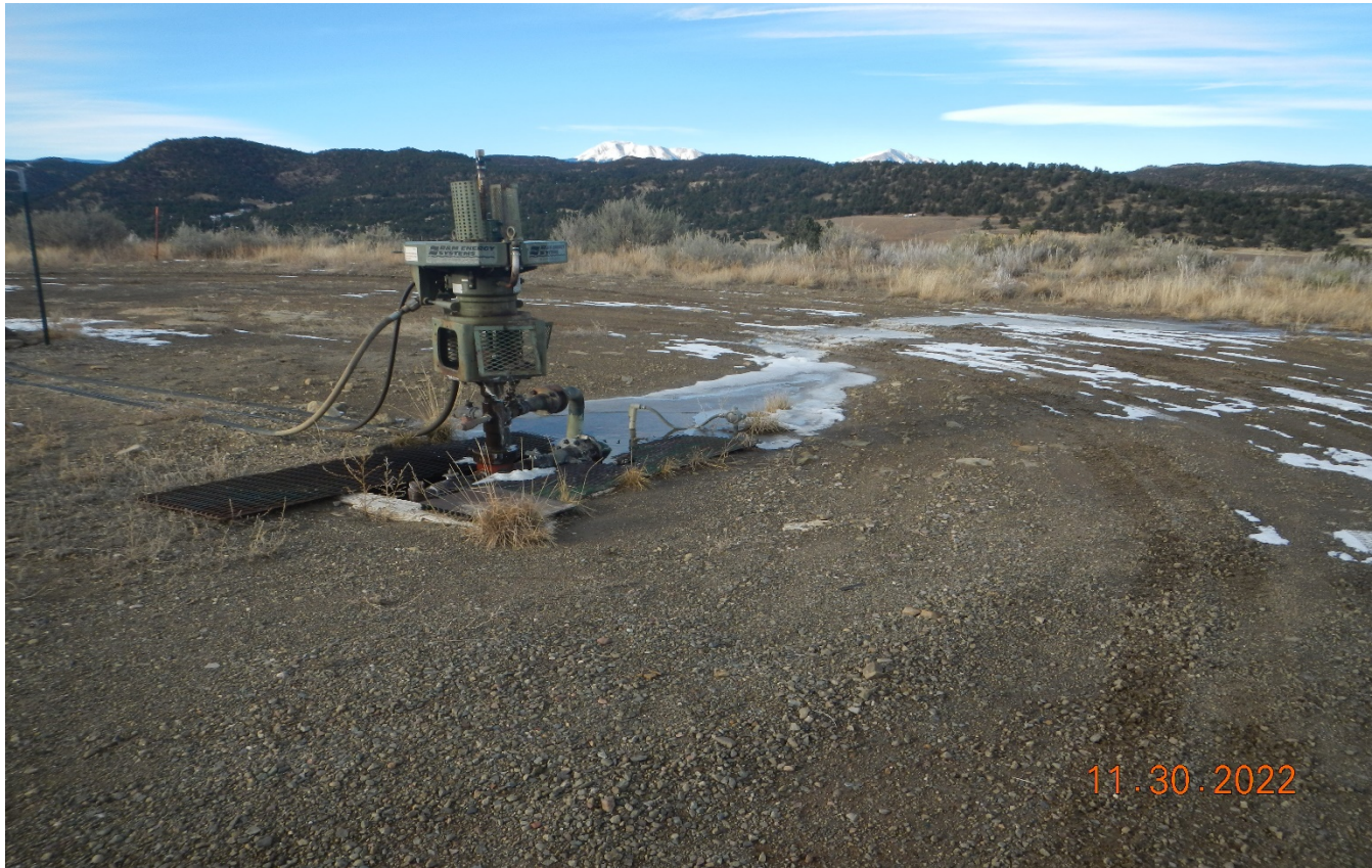
Photo 3. There is a dripping water leak at the wellhead that needs to be repaired.
