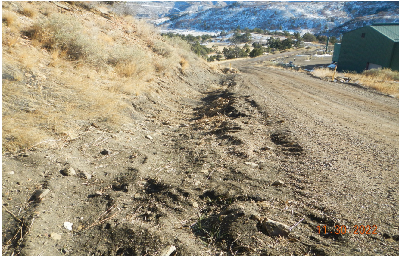
Photo 4. Further up the road. The loose soils on the roadside should be seeded for stabilization.
