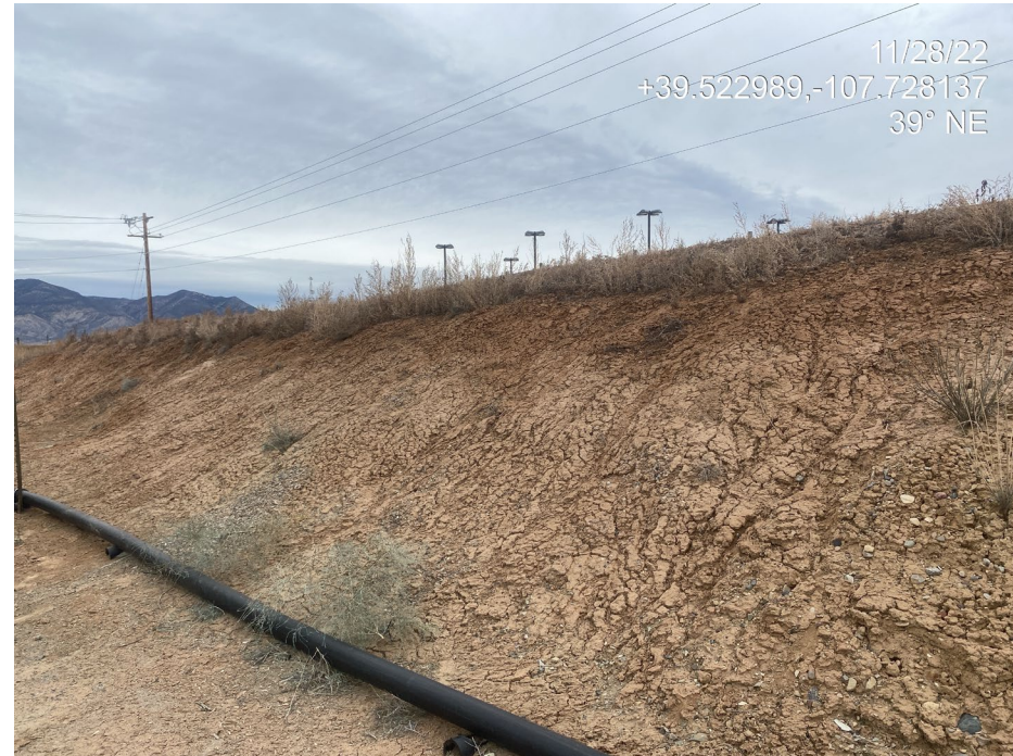
Photo 2. Photos taken from the east of the Location shows erosion occurring on cut slopes.
