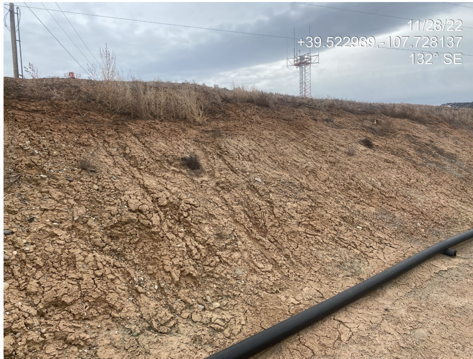
Photo 2. Photos taken from the east of the Location shows erosion occurring on cut slopes.
