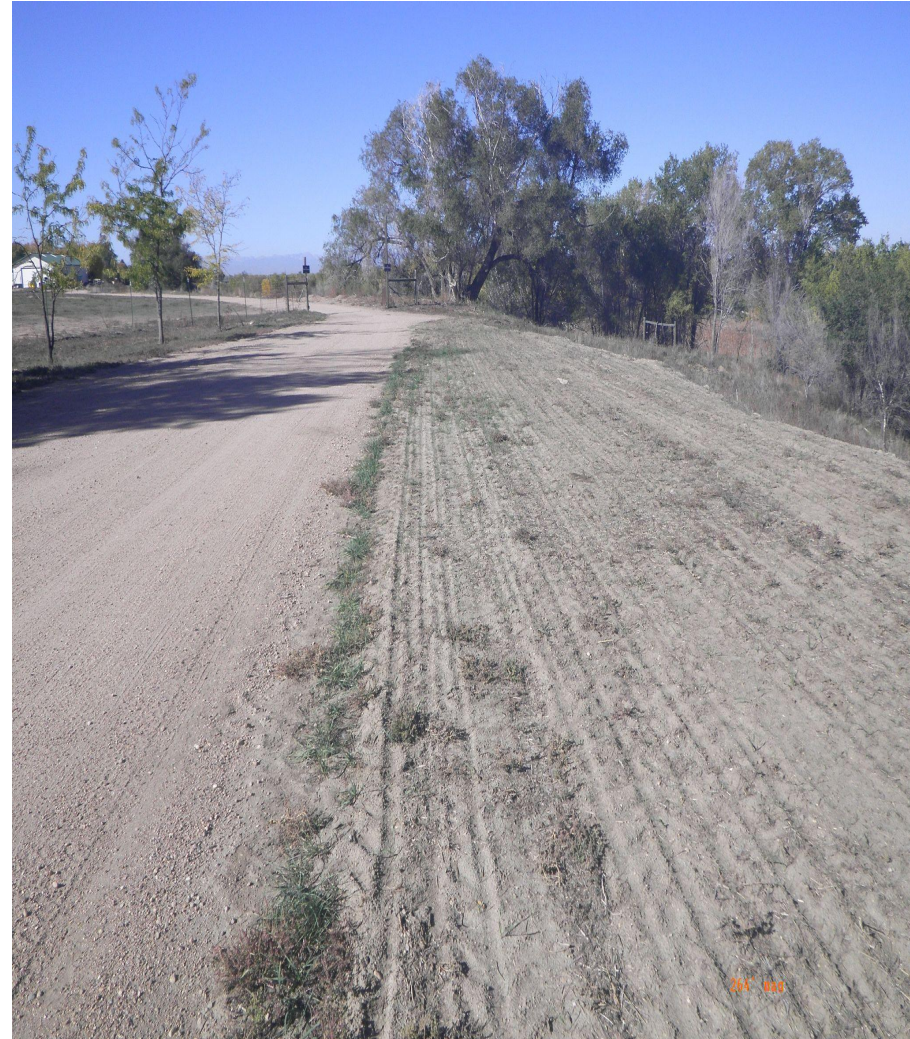
Photo 9. Cardinal photos taken at ground level from the middle of the tank battery. Left photo facing south, right photo facing west. Note: Northern portion of the tank battery has been seeded. The area has not reached the 80% threshold so the tank battery will remain in-process until the site can be re-inspected.
