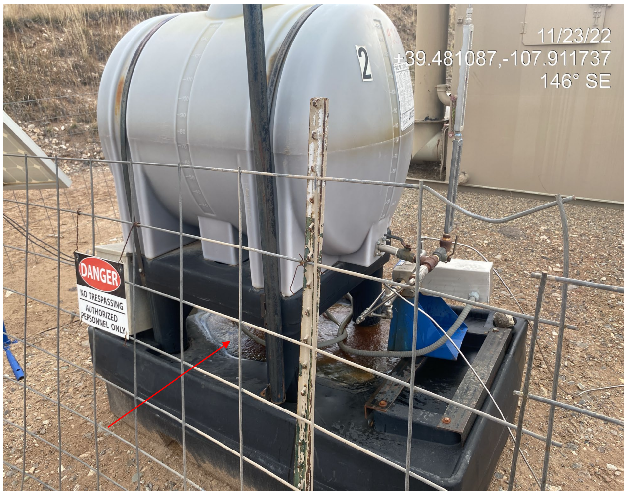
Photo 1. Photo shows a leaking corrosion inhibitor tank.
