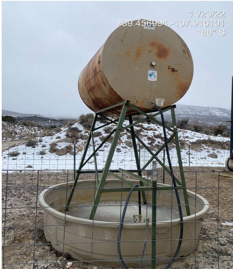
Photo 5. Photos show two secondary containment tanks lacking wildlife protection BMPs.
