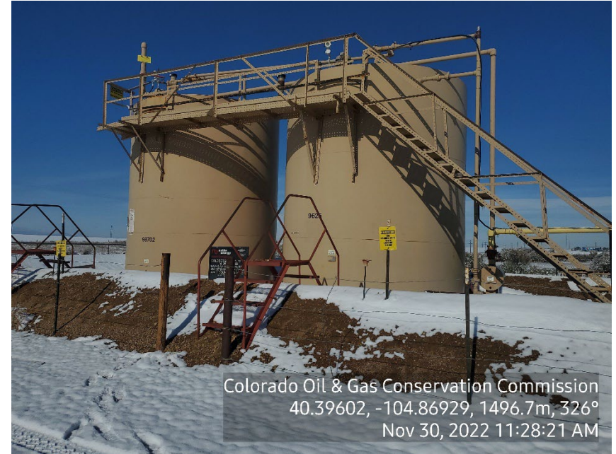
Photo 2: Tank Battery
