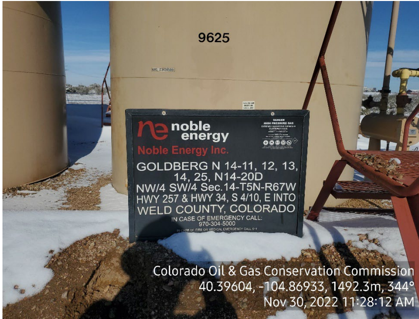
Photo 1: Tank Battery Sign
