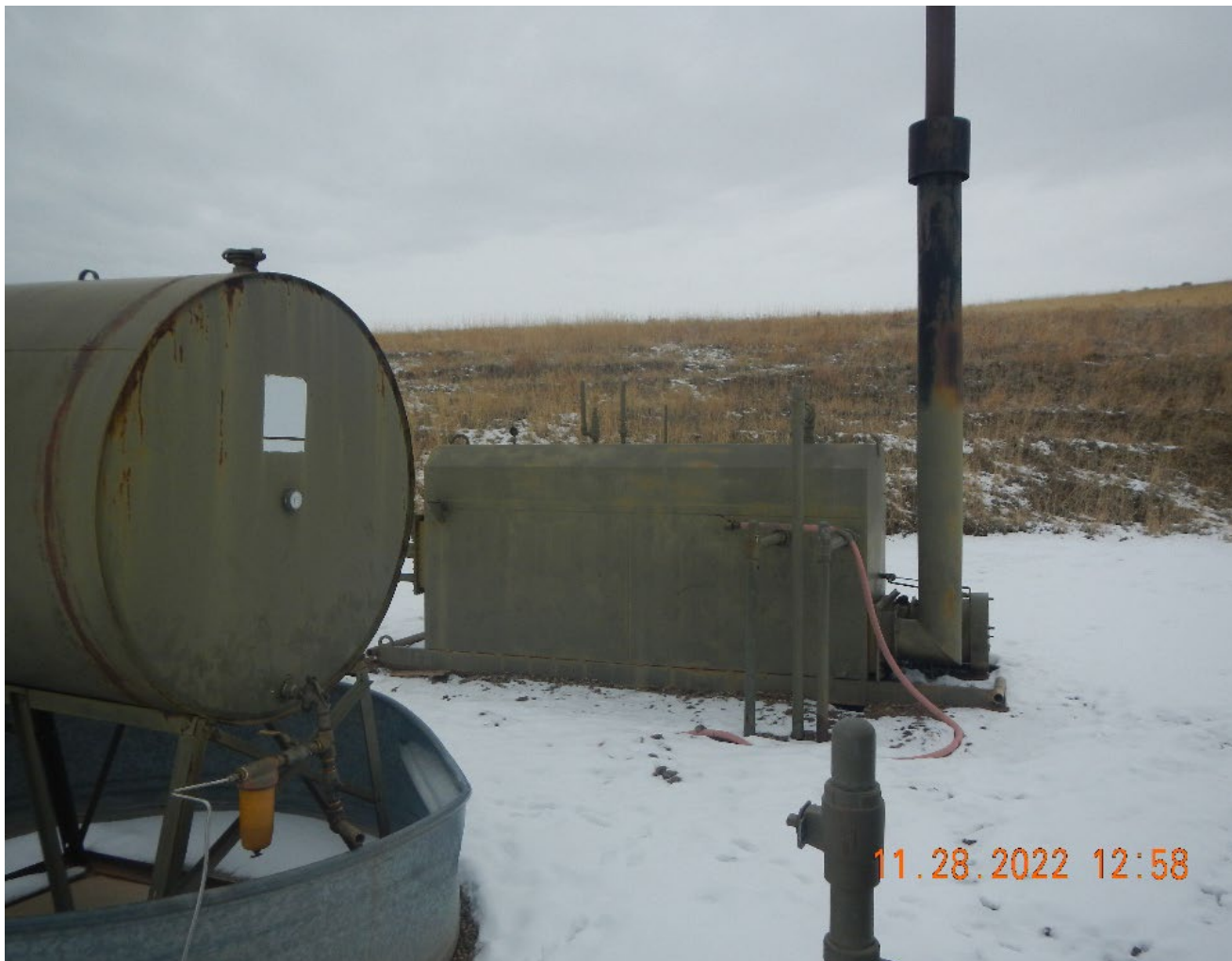
Photo #2 Dehy and unlabeled tank. No fluid was observed in the 2 nd containment. Per Rule 605.h.(3), the tank must be labeled per, "U.S. Department of Transportation's Hazardous Materials Regulations "
