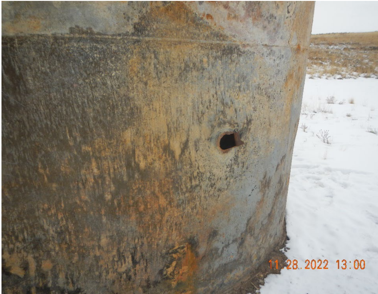
Photo #7 Penetration in tank at approximately 2 feet below ground surface.
