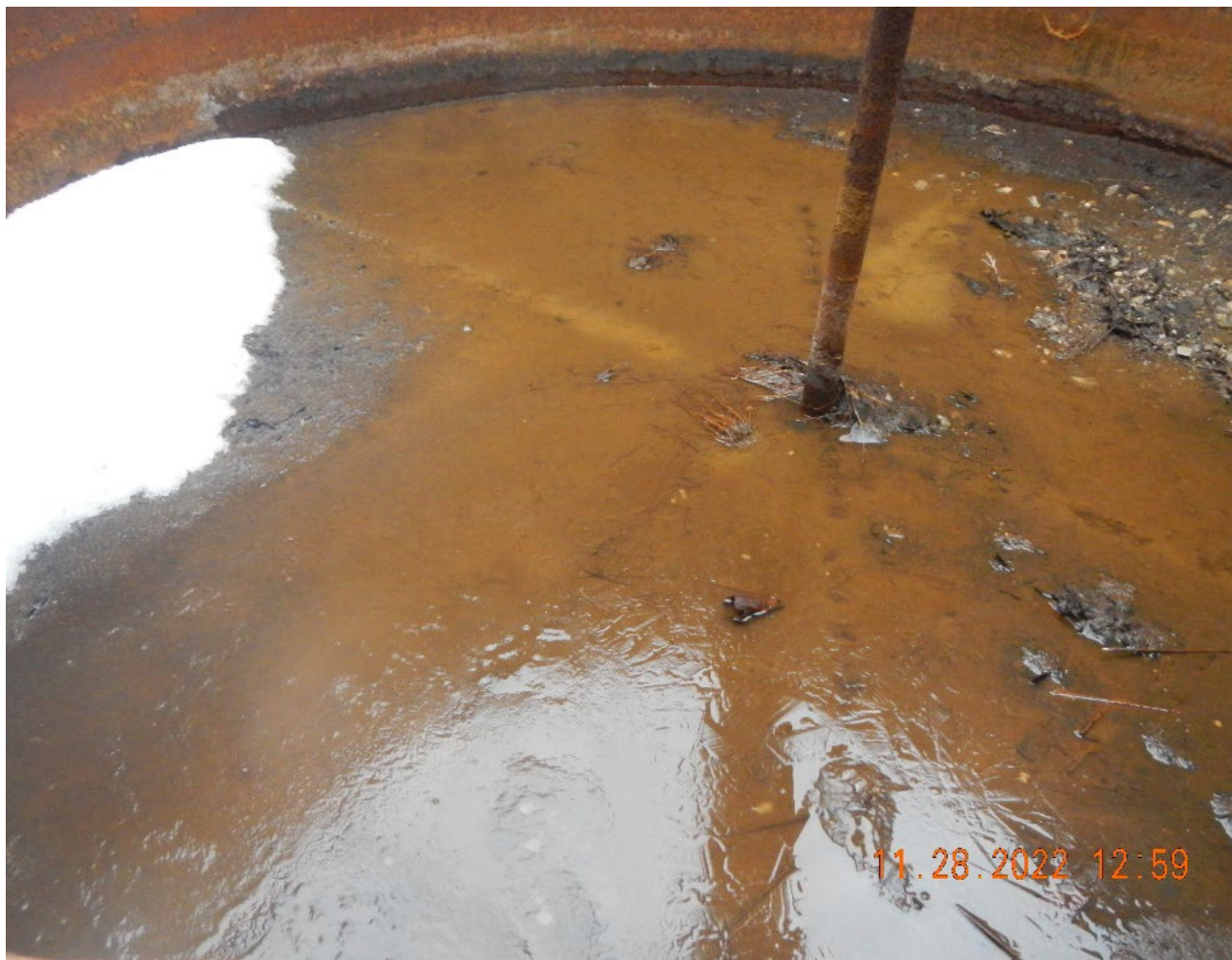
Photo #6 looking inside tank, through penetrations seen in Photo #4. There was some solids in tank, snow and fluid.
