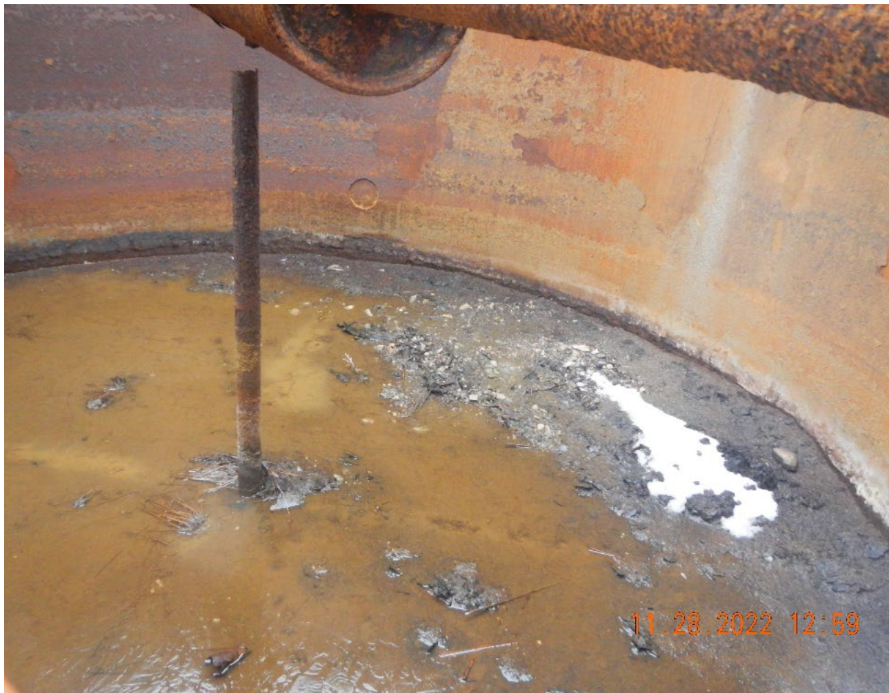
Photo #5 looking inside tank, through penetrations seen in Photo #4. There was some solids in tank, snow and fluid.
