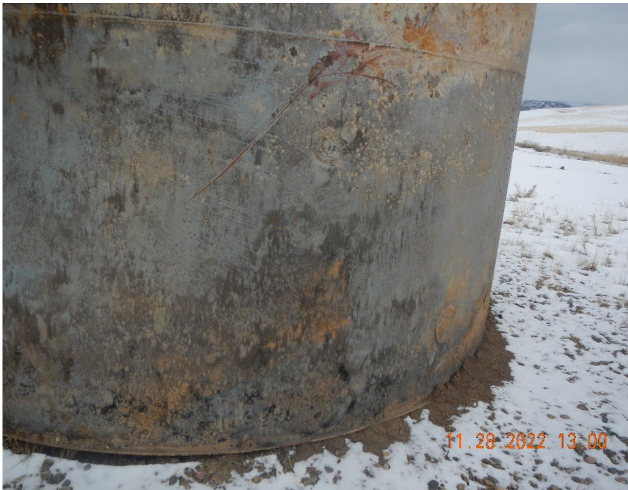
Photo #8 Close up of tank condition. The tanks location, when in service is identified in Photo #11 as, “partially buried vessel”.
