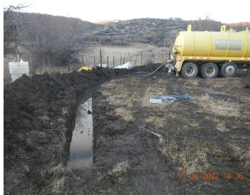
Initial response containment berm and collection area for released fluids.
