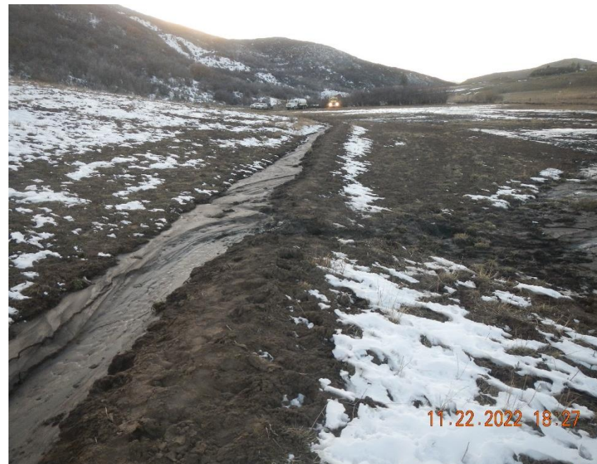
Area where released fluids breached the bank of a storm water diversion ditch.
