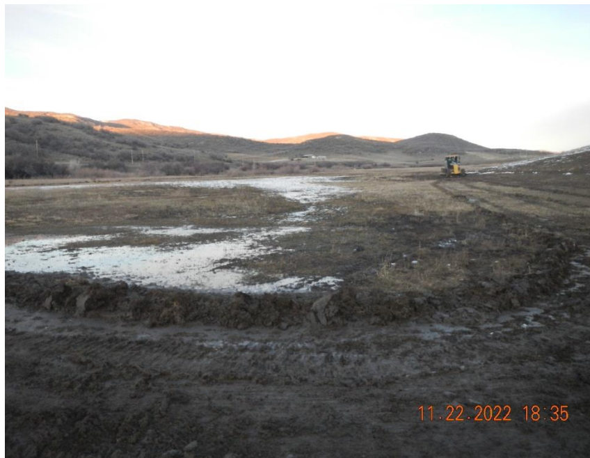
Affected field with grader creating a containment berm.
