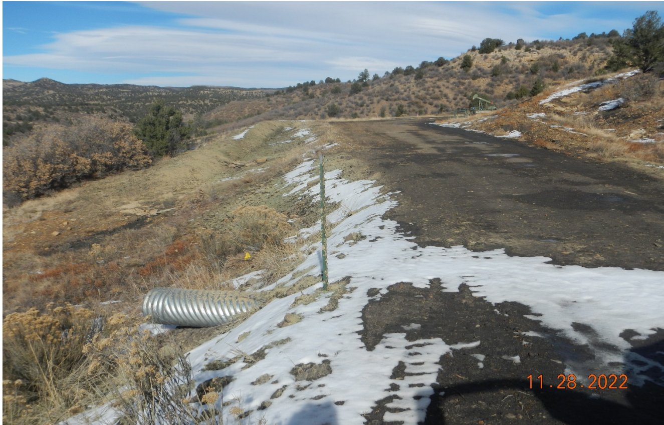
Photo 2. The erosion along the access road has been repaired.
