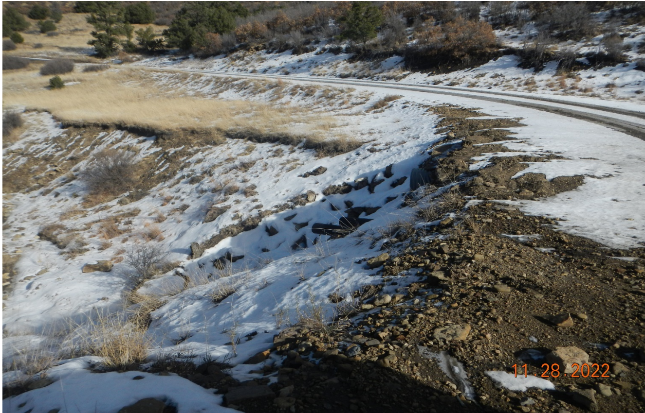
Photo 1. There has been outlet protection installed at the culvert outlet.
