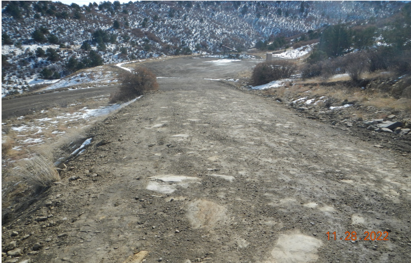
Photo 4. Facing southeast toward the well site.
