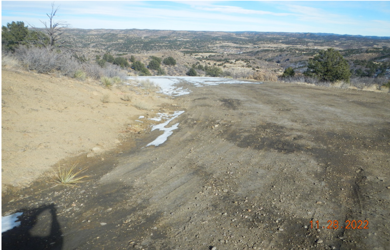
Photo 1. Facing north toward the beginning of the access road. The road side was hydromulched and seeded..
