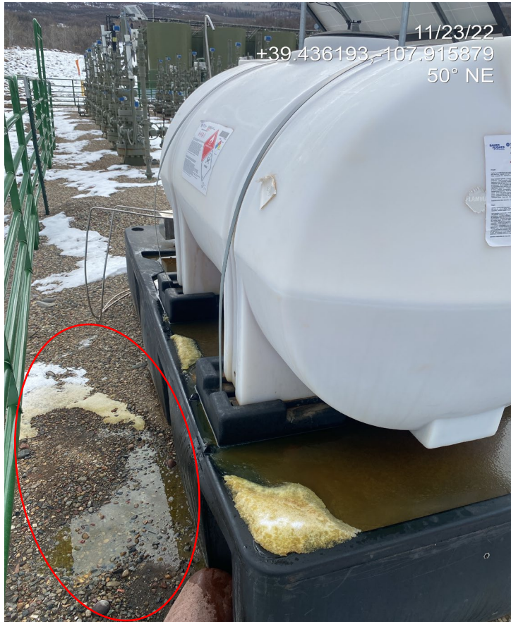
Photo 2. Photo taken from the well area shows one of two leaking corrosion inhibitor tanks. Fluid observed outside secondary containment on the ground.
