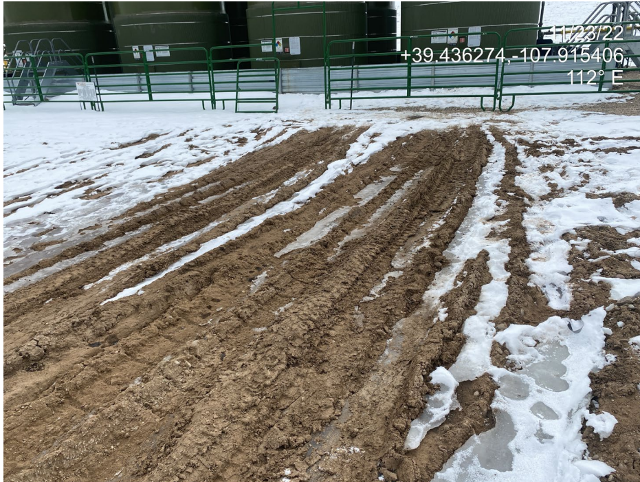
Photo 9. Photo shows compaction and gravel degradation of pad surface.
