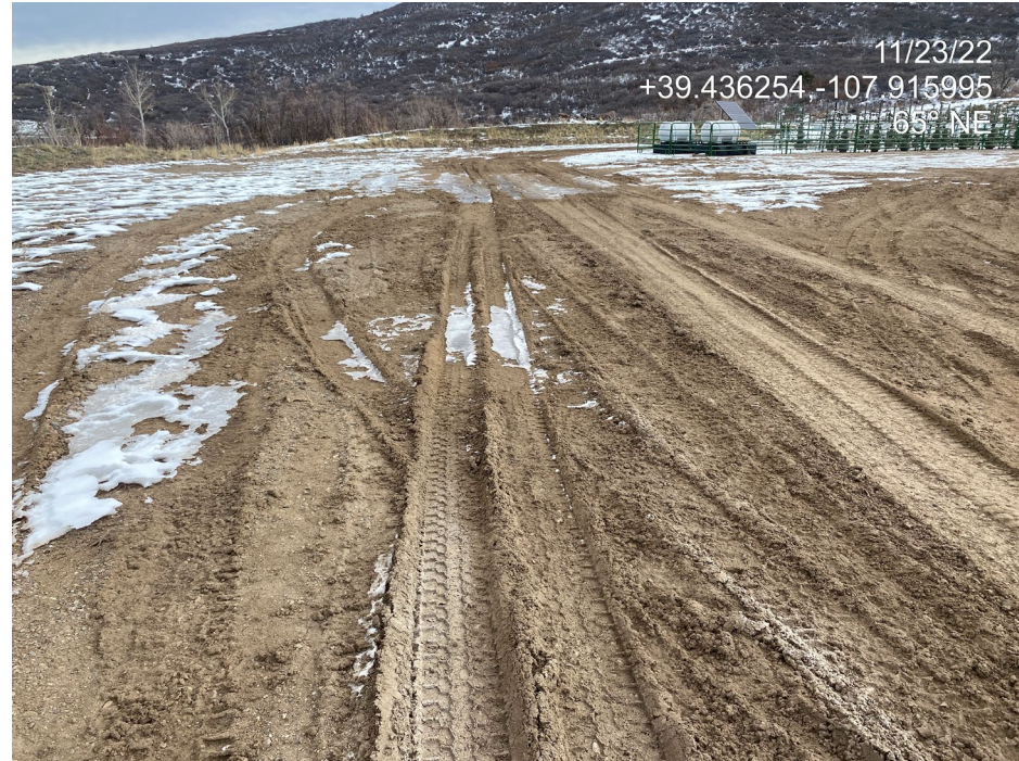
Photo 10. Photo shows compaction and gravel degradation of pad surface
