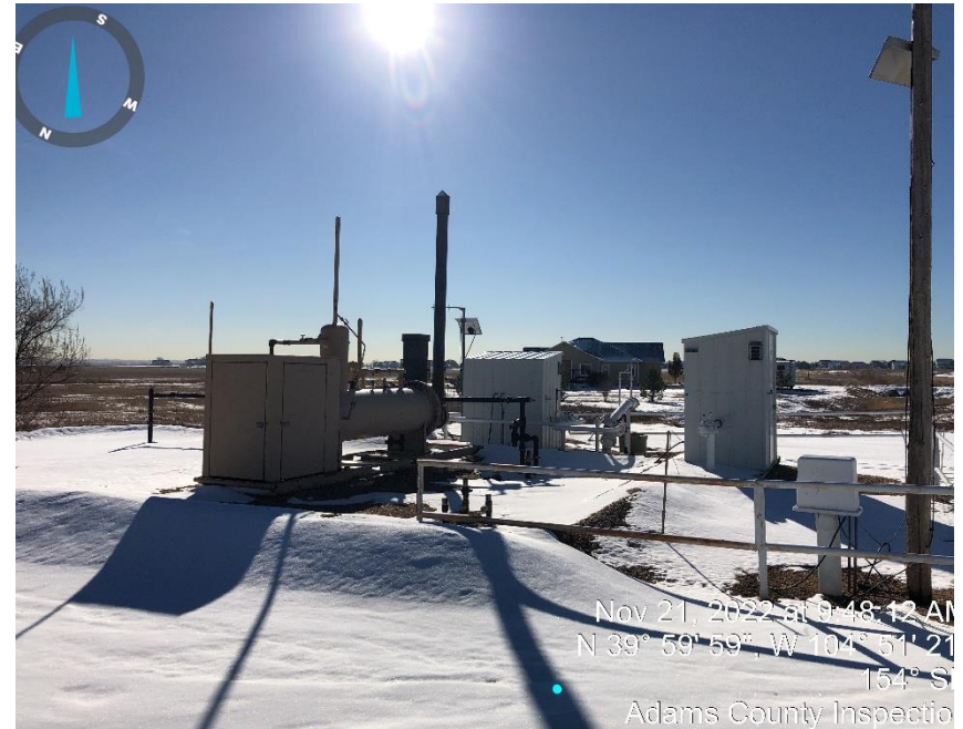
Photo#2 Meter runs, Separator and ECD.
