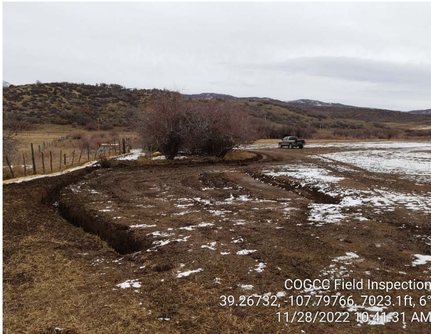
Photo #9 – View of recovery trenches at northwest end of flow path, looking north.
