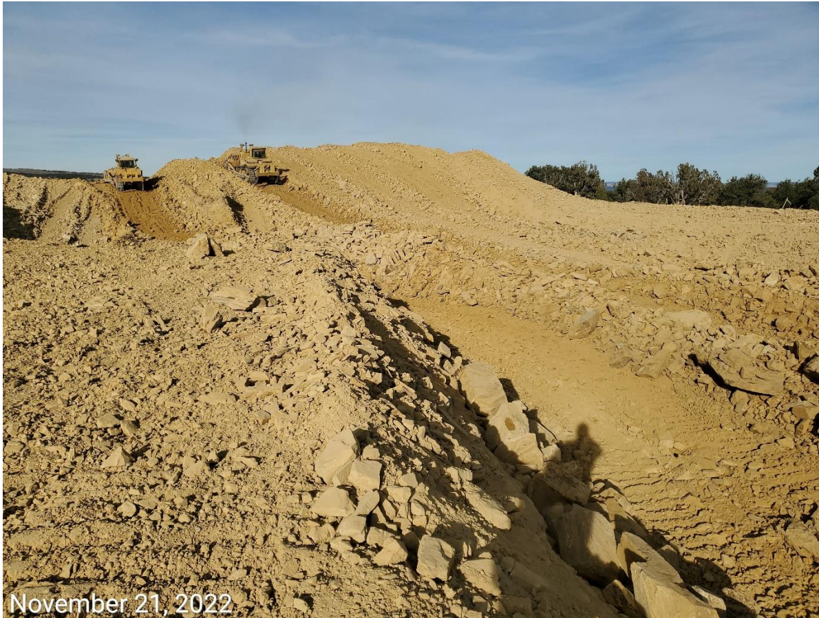
Photo 7: Photo shows construction of the cuttings trench “in process”.
