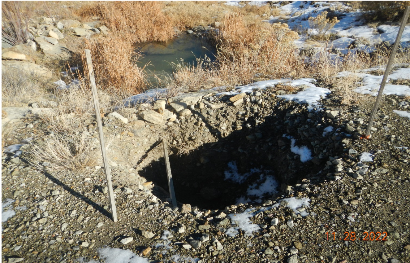
Photo 2. There is a hole in the culvert at the drainage crossing causing material to cave in in this area of the road.
