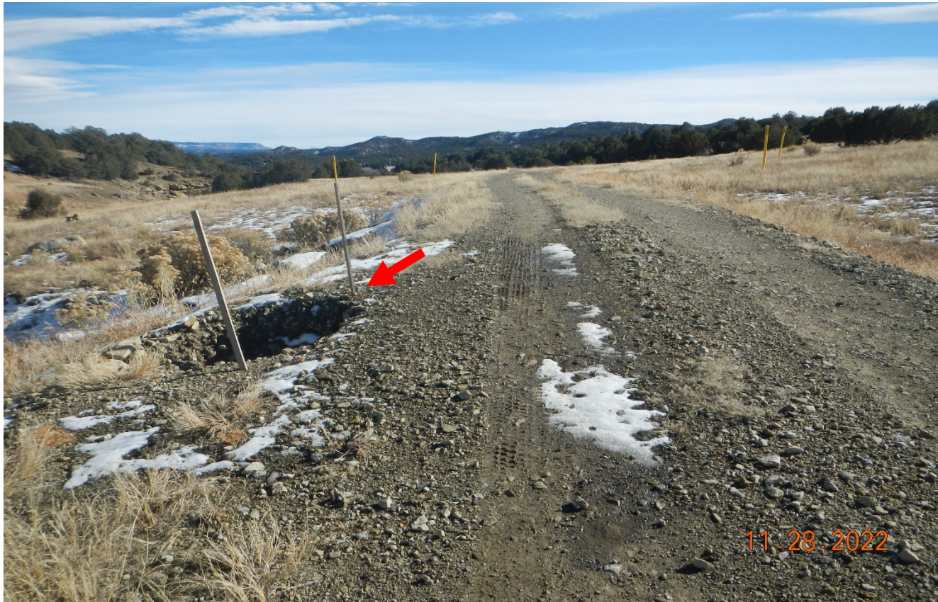
Photo 1. Facing southeast along the access road. There is an open hole at the culvert crossing that needs to be repaired.
