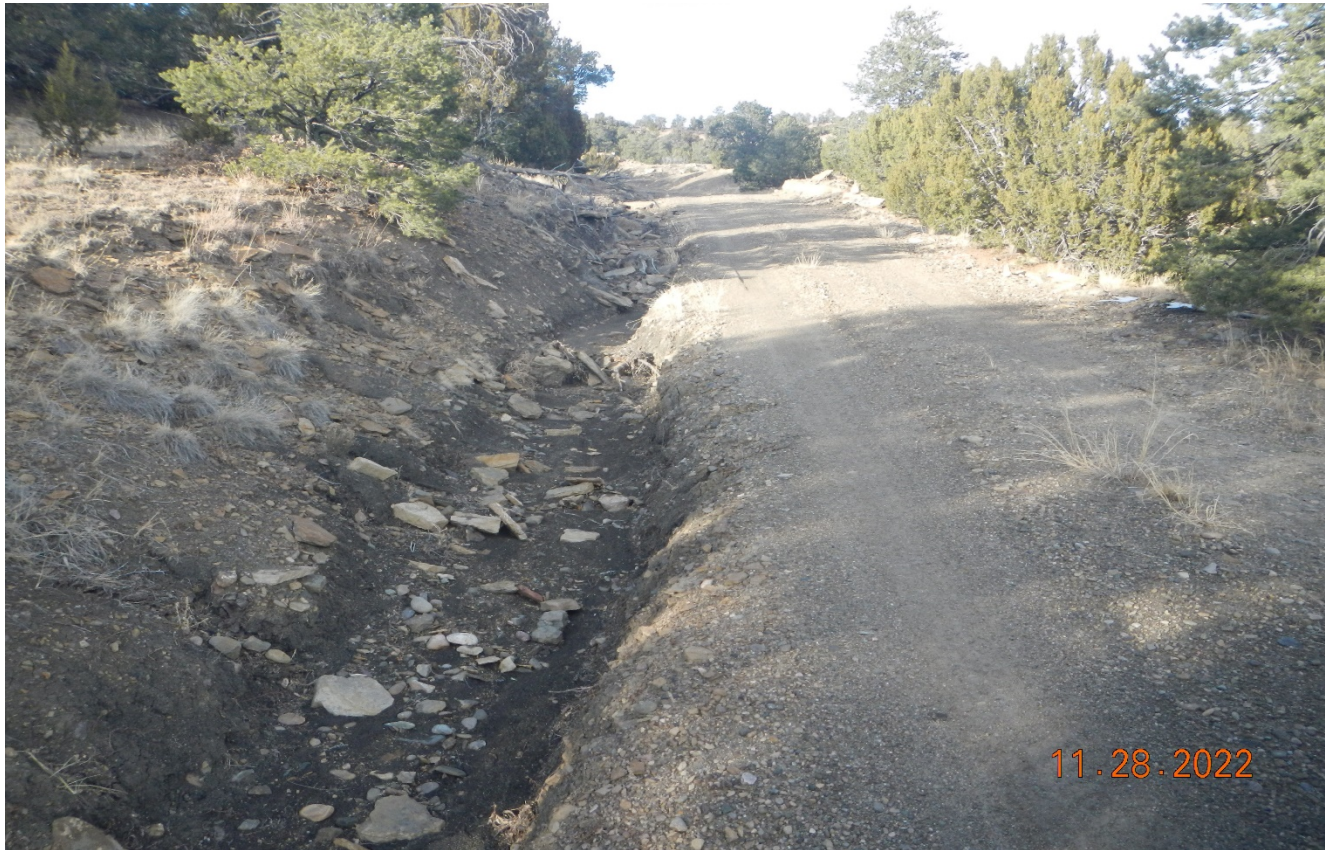
Photo 1. Facing north along the access road. There is erosion along the roadside that needs to be repaired with BMP's
