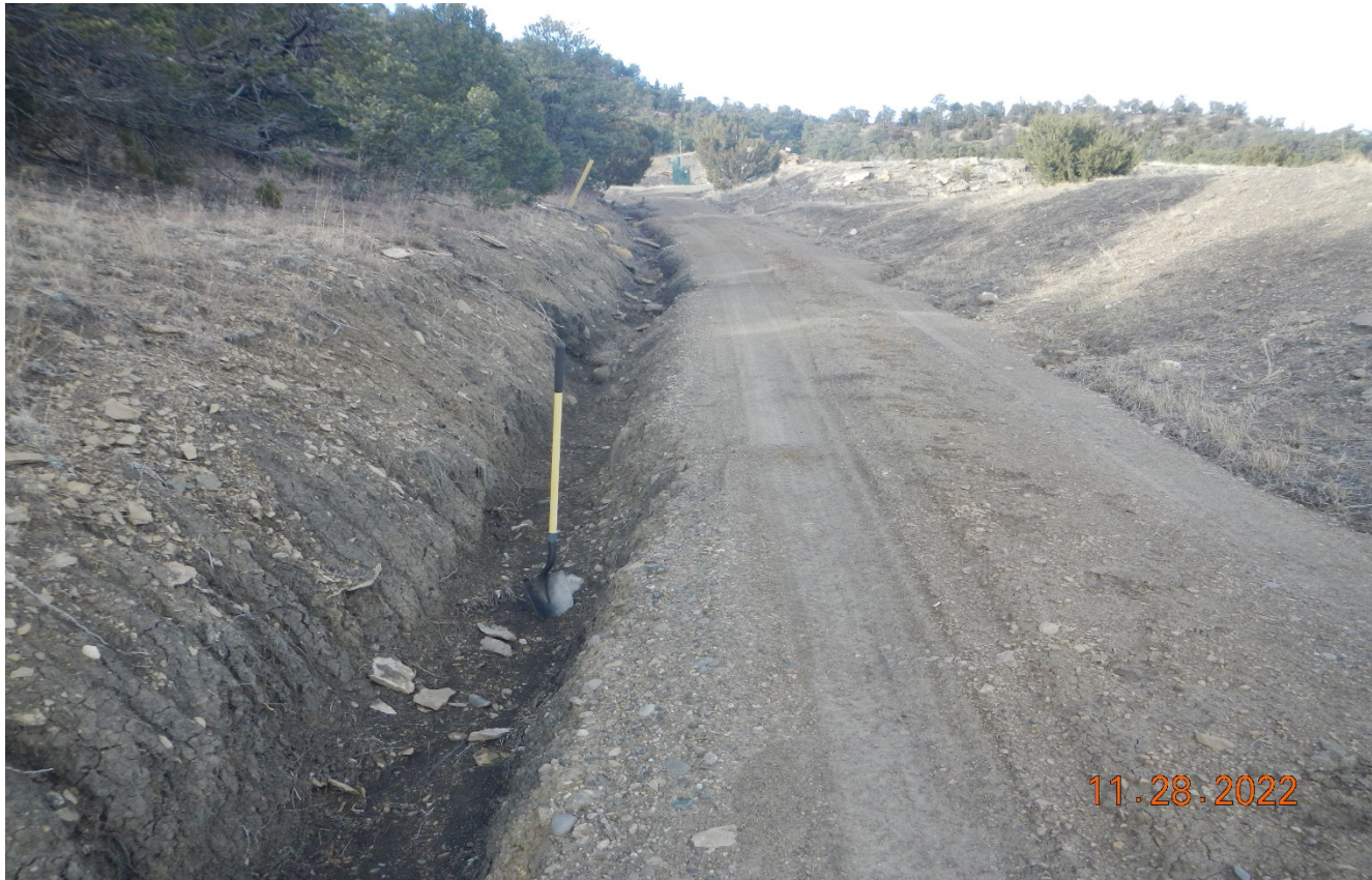
Photo 2. Facing north along the access road. There is erosion along the roadside that needs to be repaired with BMP's
