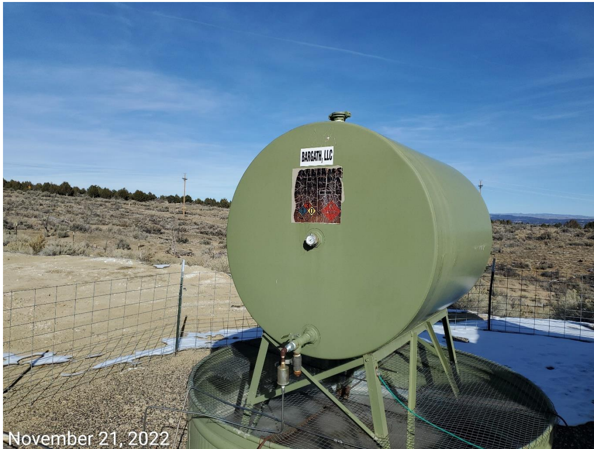
Photo 4: Photo of tank adjacent to the separator equipment. Photo shows label information is illegible. Operator information also incorrect.
