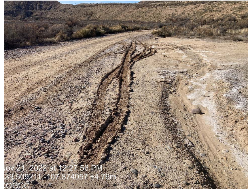
Lack of stabilization/ compaction
