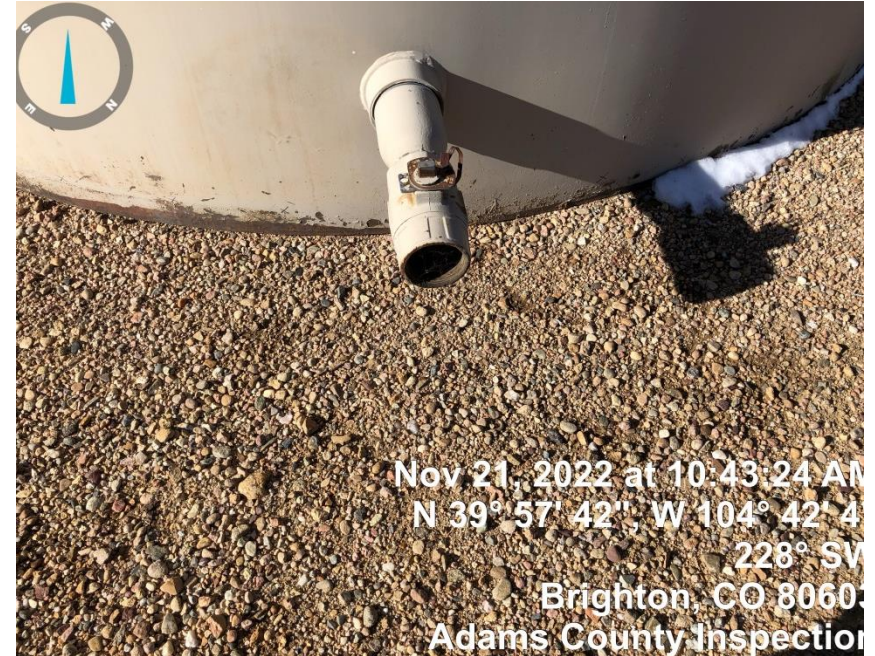
Photo#4 Corrective Action: No bull plug on Load out line
