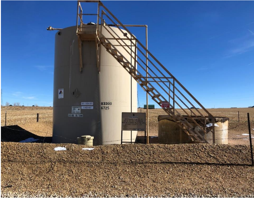
Photo#1 Production Tank/Produced Water Tank
