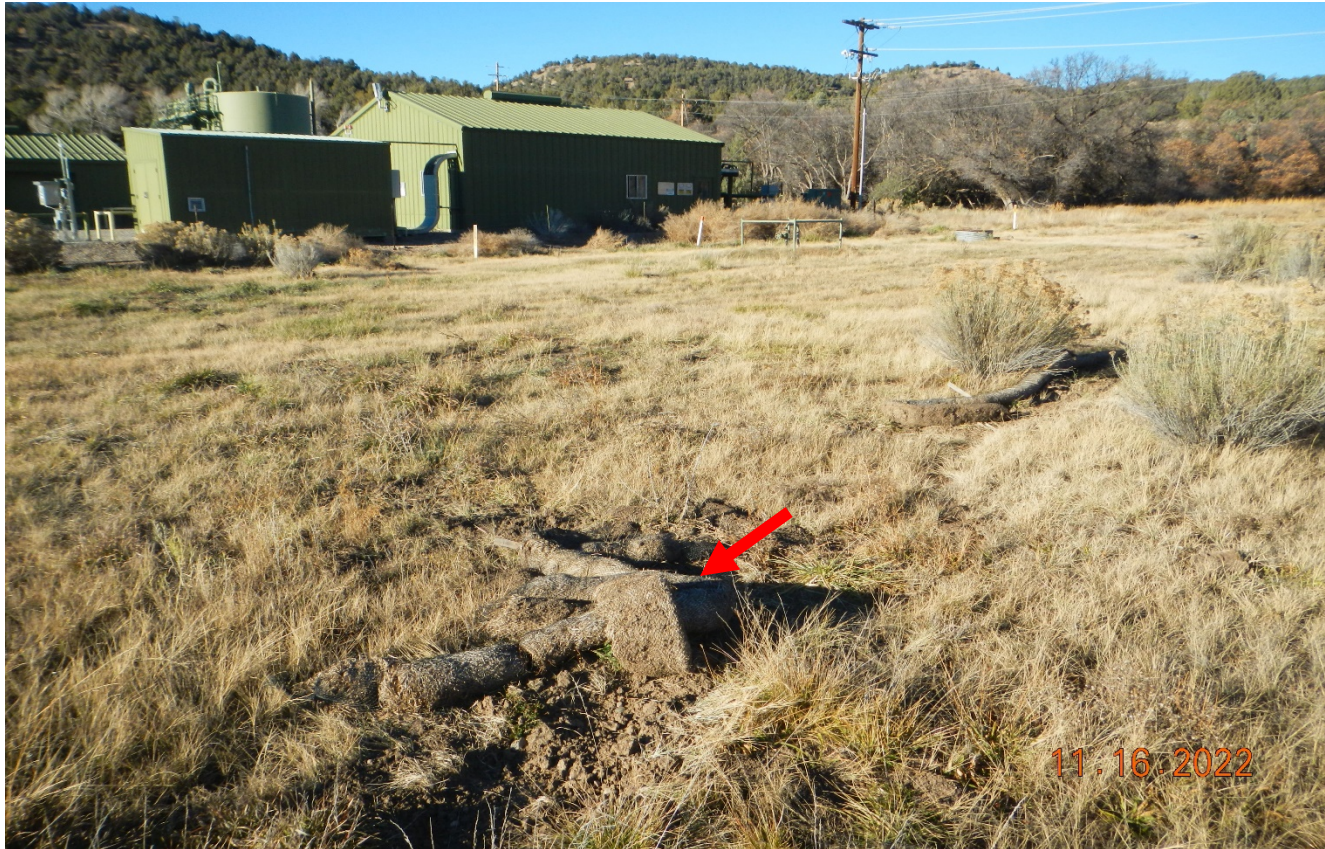
Photo 2. Facing northeast at the location. There are displaced wattles that need to be removed.
