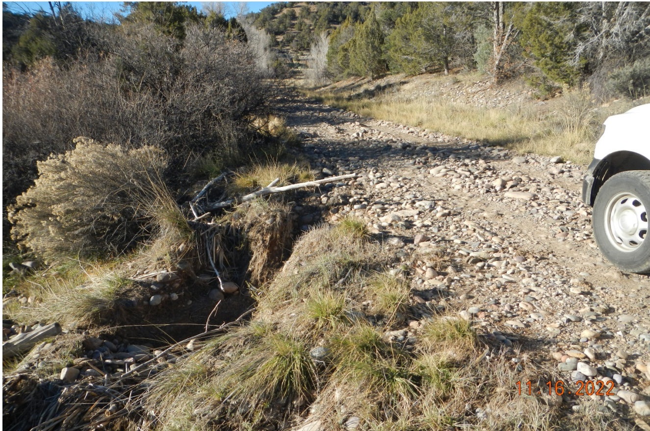
Photo 4. Facing northwest along the access road. There is vehicle rutting and erosion along the road that needs to be repaired. Stormwater further up the drainage is being directed down the road to this area.
