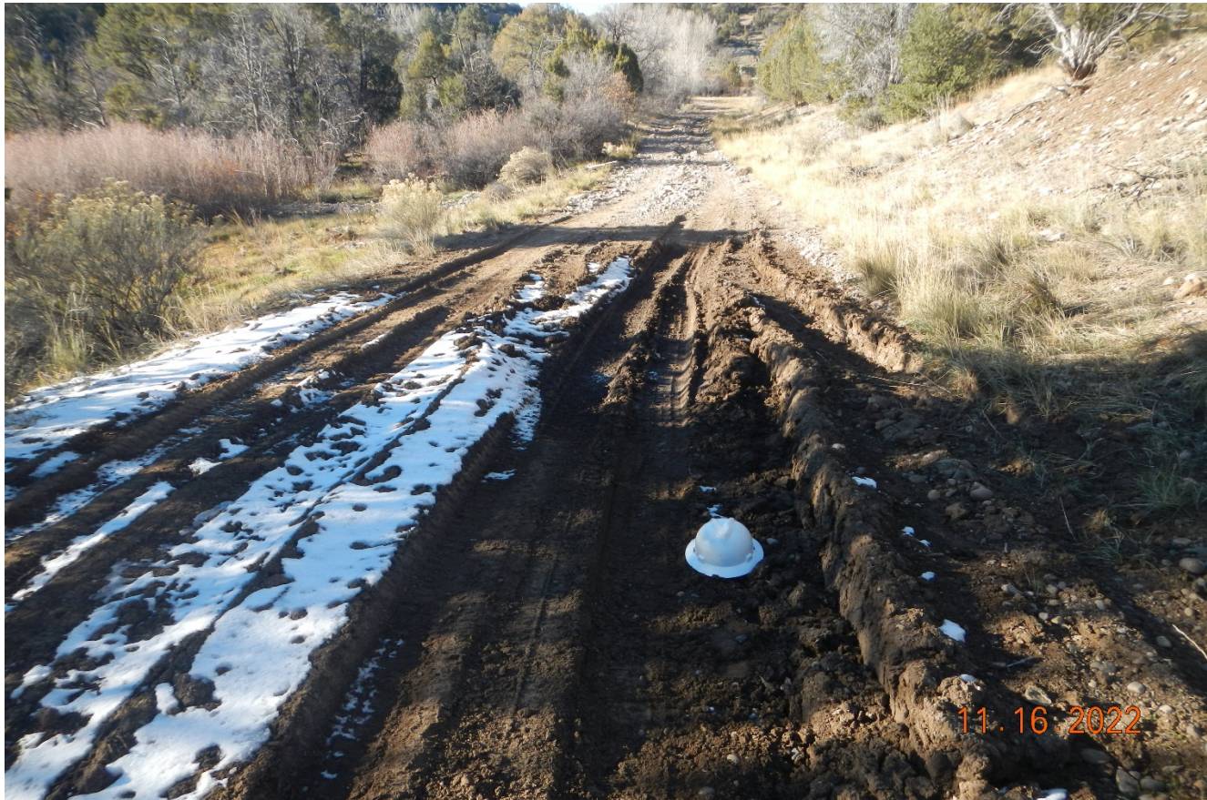
Photo 3. Facing northwest along the access road. There is vehicle rutting and erosion along the road that needs to be repaired. Stormwater further up the drainage is being directed down the road to this area.
