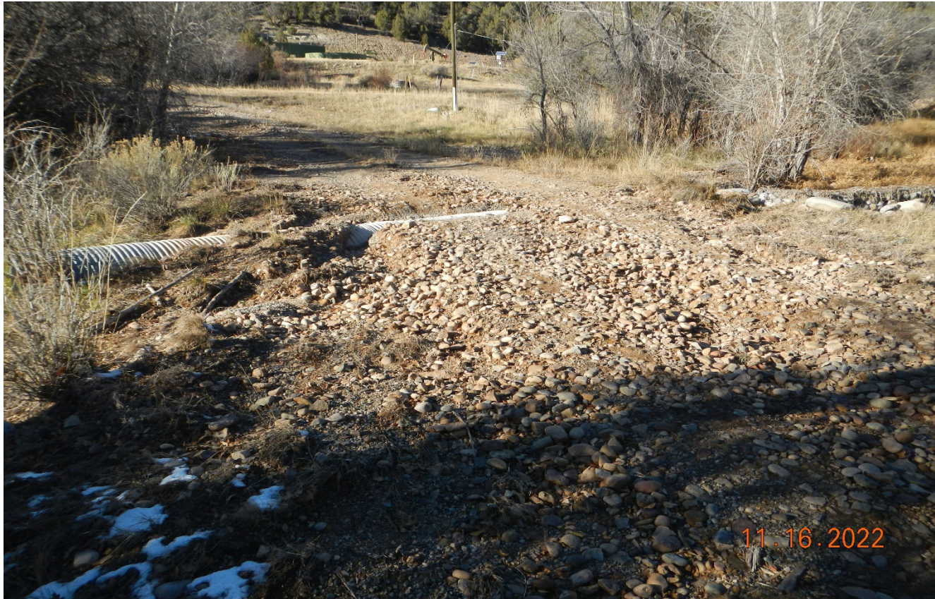
Photo 5. Stormwater from the drainage at right side of photo is being directed down the road and has washed out this culvert due to insufficient size of culvert. A larger or multiple culverts are needed to allow proper drainage away from the road. Lat/Long:37.13507,-107.83293.
