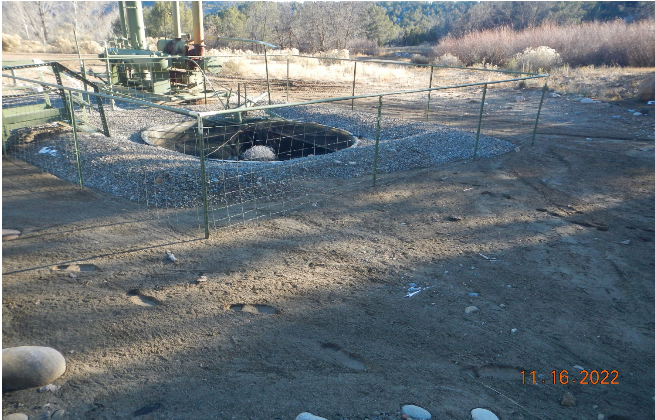
Photo 7. Facing toward the open top tank. Sediment has accumulated at the berm of the tank and stormwater is being directed into the tank. Stormwater needs to be divert away from the open top tank and berm repaired.
