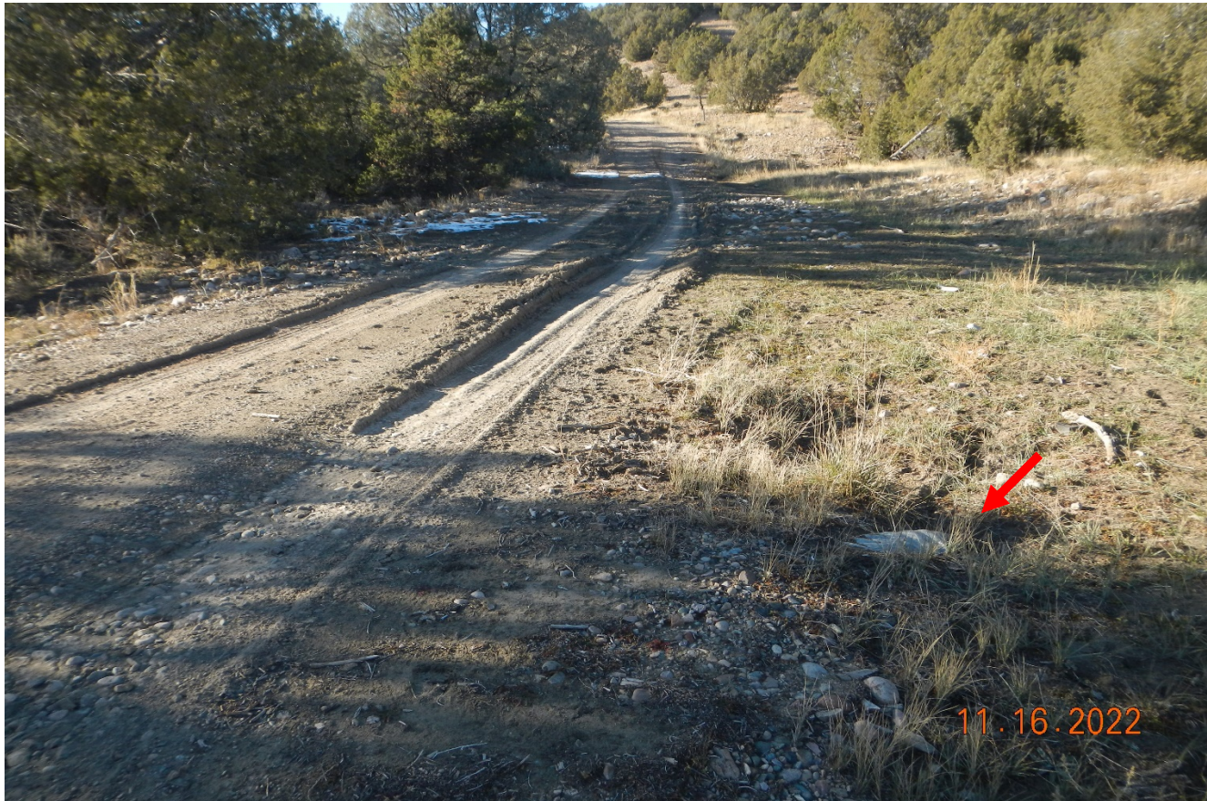
Photo 2. Stormwater is not being directed toward the culvert at red arrow which is causing erosion of the road. Lat/Long:37.13286,-107.82855
