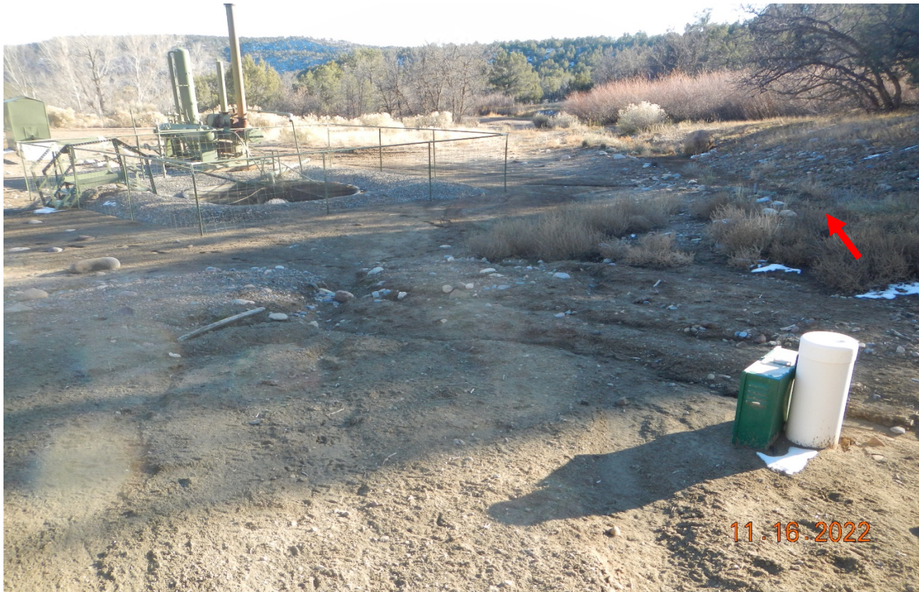
Photo 8. Northwest side of the location facing southwest. The diversion ditch at red arrow has filled in with sediment causing stormwater and sediment to flow toward the open top tank.
