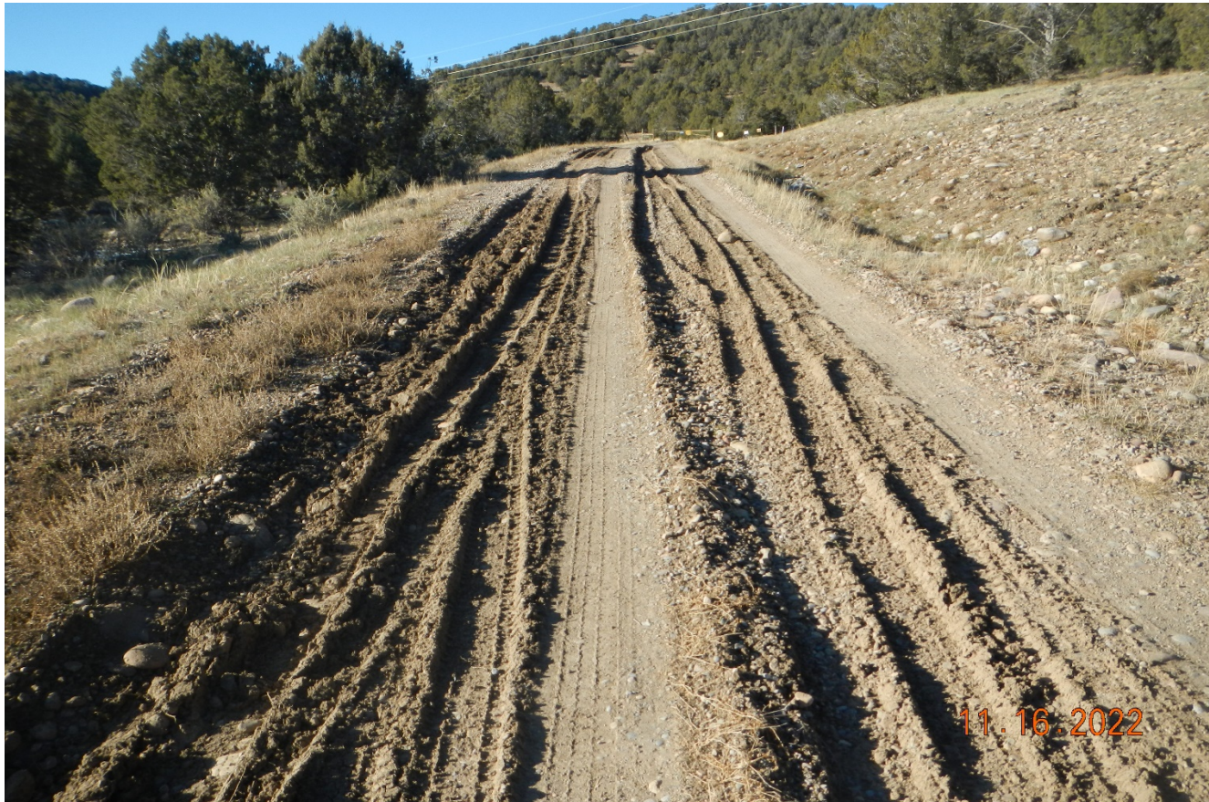
Photo 1. Facing northwest along the access road. There is vehicle rutting and erosion along the road that needs to be repaired.
