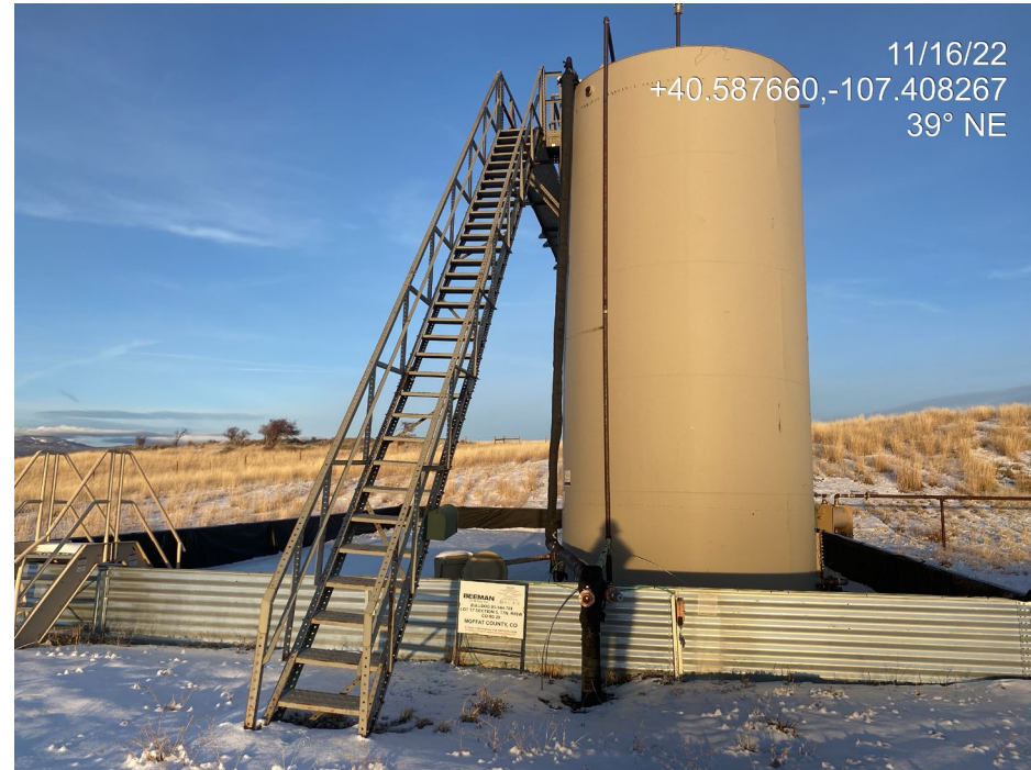
Photo 3. Photo shows a tank battery sign has been installed. Sign does not comply with Rule 605.e; API number absent.
