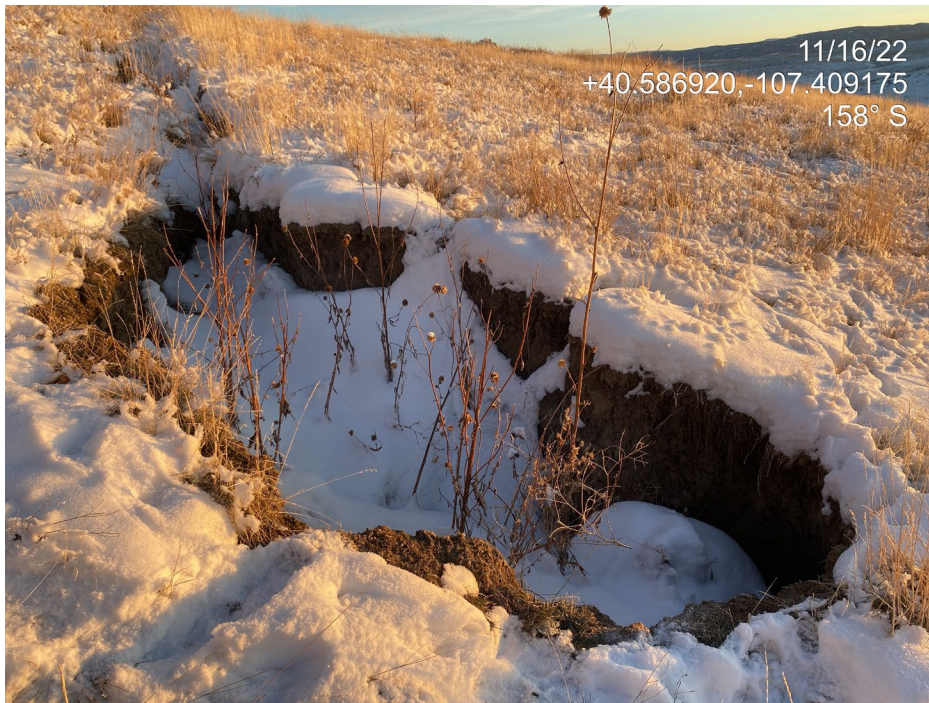
Photo 8. Photo taken from the west of the Location shows where a stormwater ditch is eroding and forming a gully. The gully is expanding and eroding downward, forming a deep hole.
