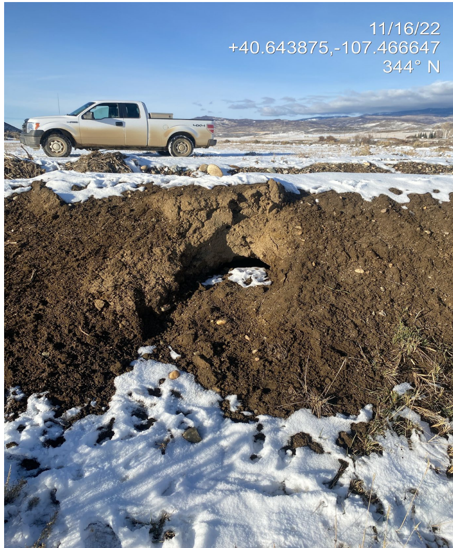
Photo 5. Photo taken from the southeast of the Location shows where the perimeter stormwater berm has been compromised and is not maintained in proper functioning condition.
