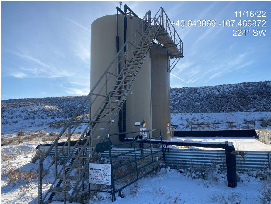
Photo 3. Photo shows the tank battery sign (left) and wellhead sign (right) both lack the well API number. Photos also show vegetation and vegetation debris around production equipment.
