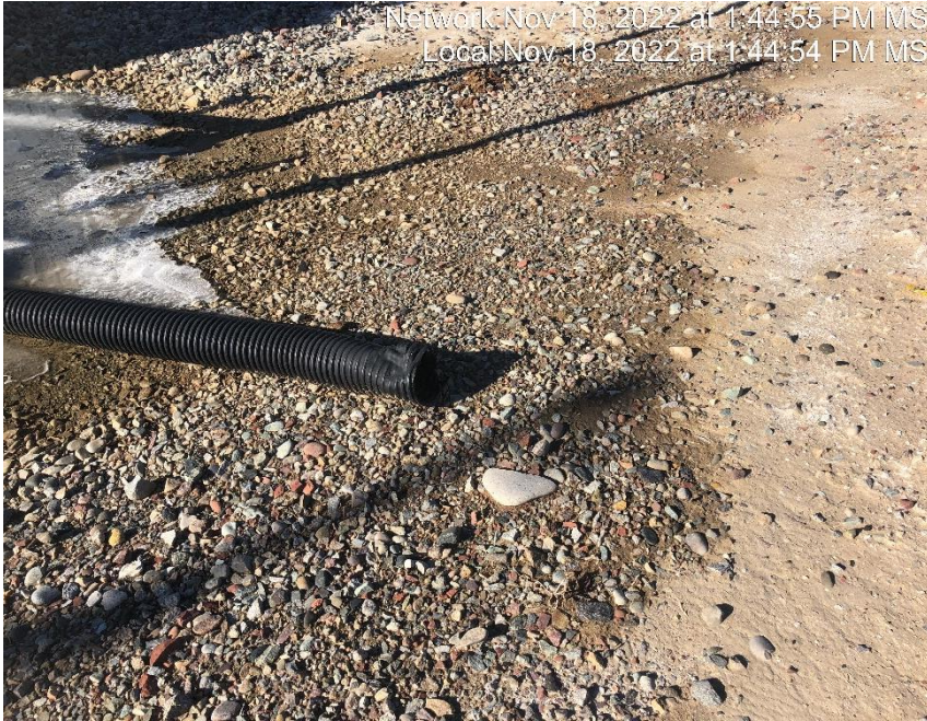
Photo #8463 Flowline heating insulation open ended.
