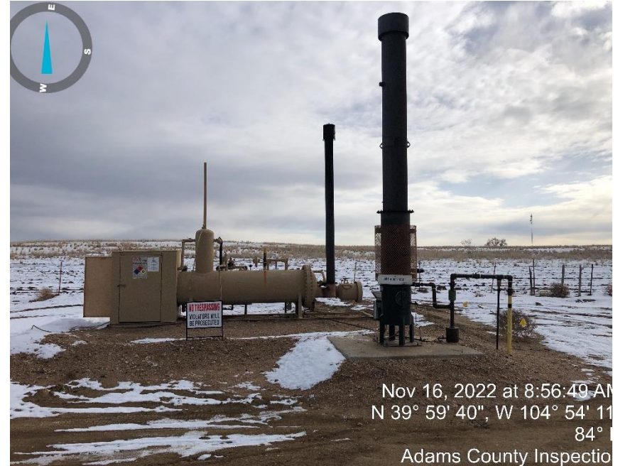
Photo#2 Separator & ECD.
