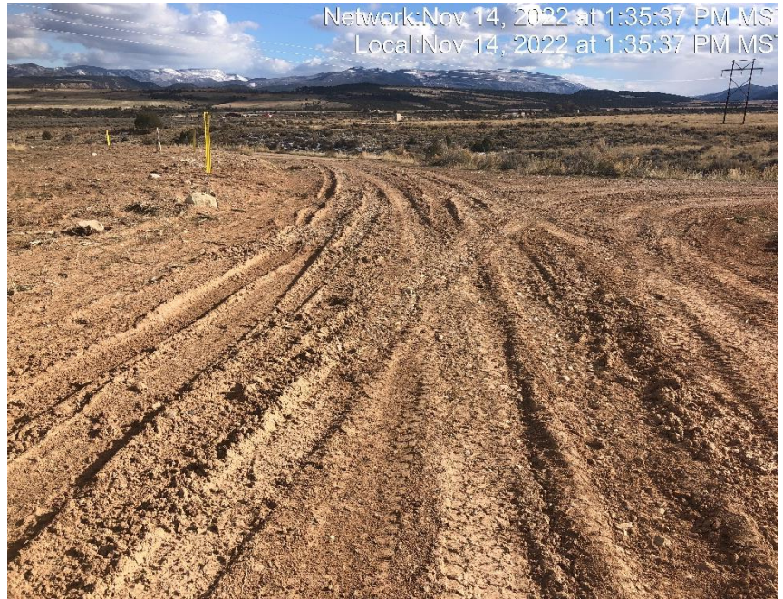
Photo #8393 Insufficient tracking control at entrance to location.
