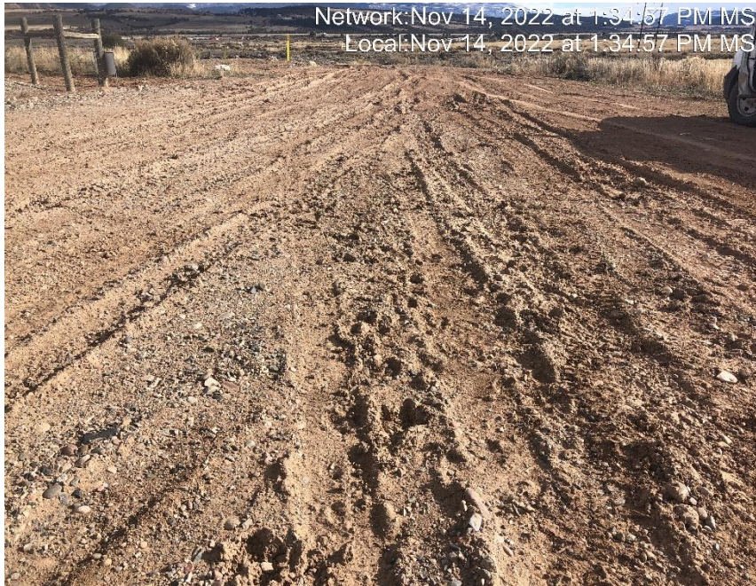
Photo #8391 Location lacks stabilization.
