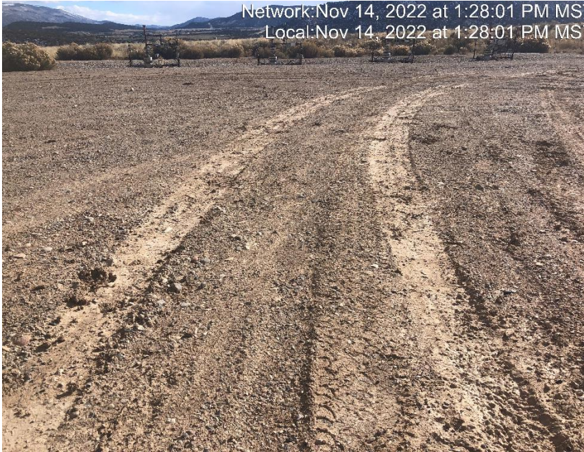
Photo #8381 Location lacks stabilization.
