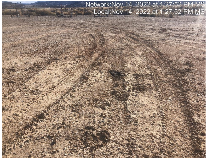
Photo #8380 Location lacks stabilization.
