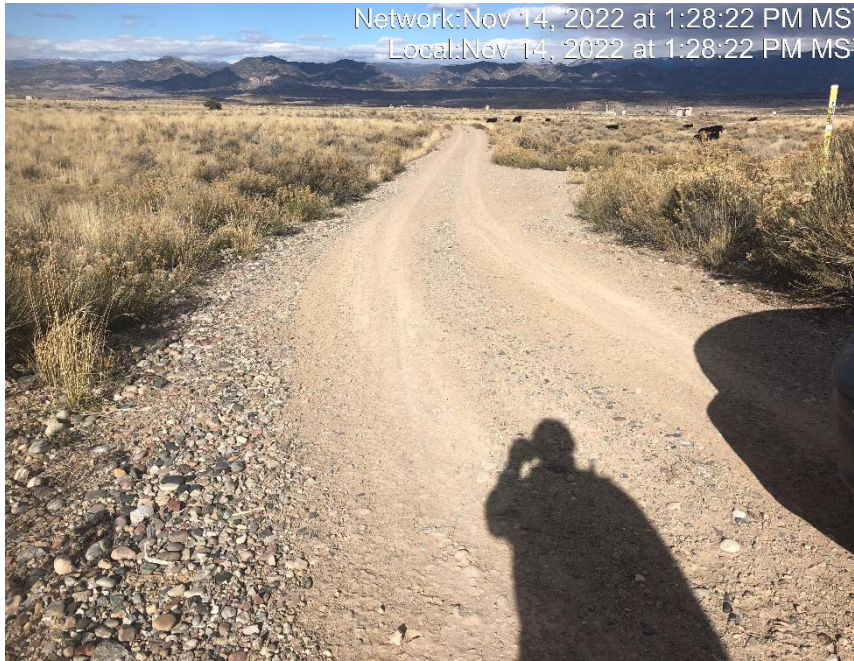
Photo #8383 Insufficient tracking BMP at entrance to location.
