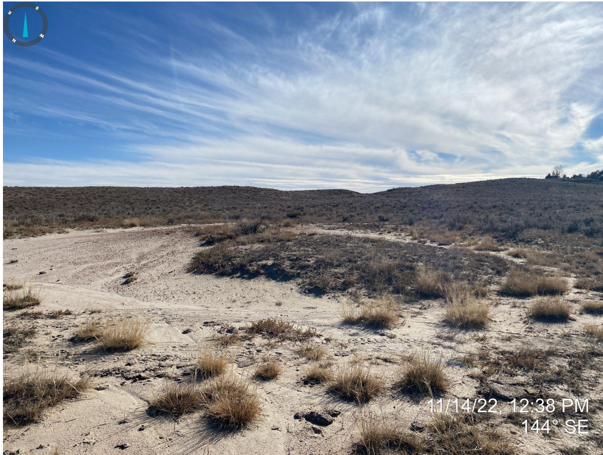
Photo 1. Taken from location, facing southeast. Photo illustrates the location has not been reclaimed with major contour and grading issues evident and areas of bare soil possibly a result of compaction issues or a possible produced water spill.
