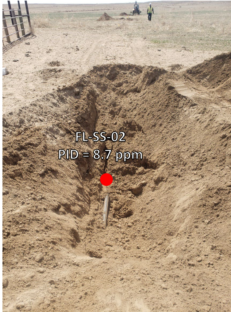
Looking south at cut point – flowline abandoned between FL-SS-01 and FL-SS-02 No petroleum hydrocarbon staining or odor observed
