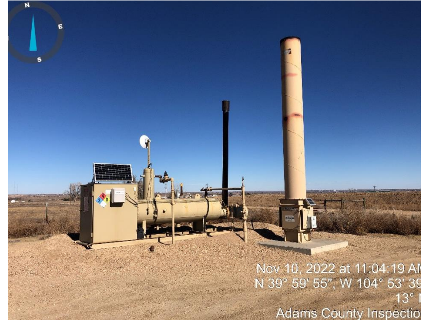
Photo#4 Separator & ECD.
