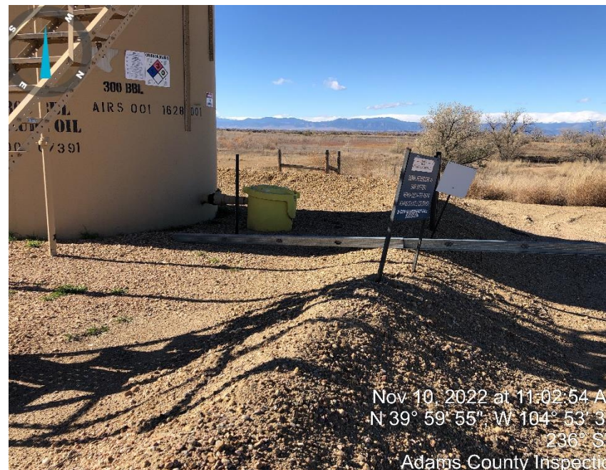
Photo#2 Crude Tank berm.
