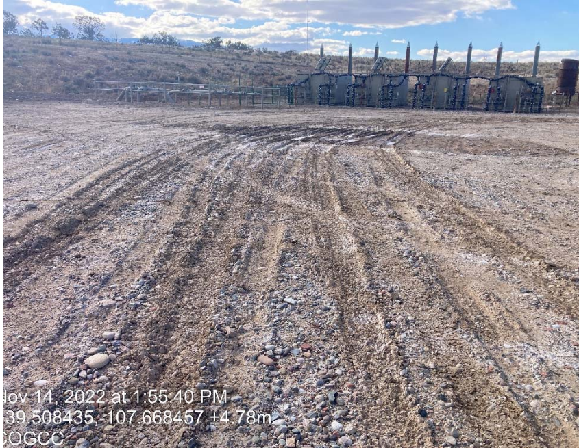
Lack of stabilization/ compaction
