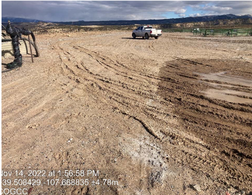
Lack of stabilization/ compaction
