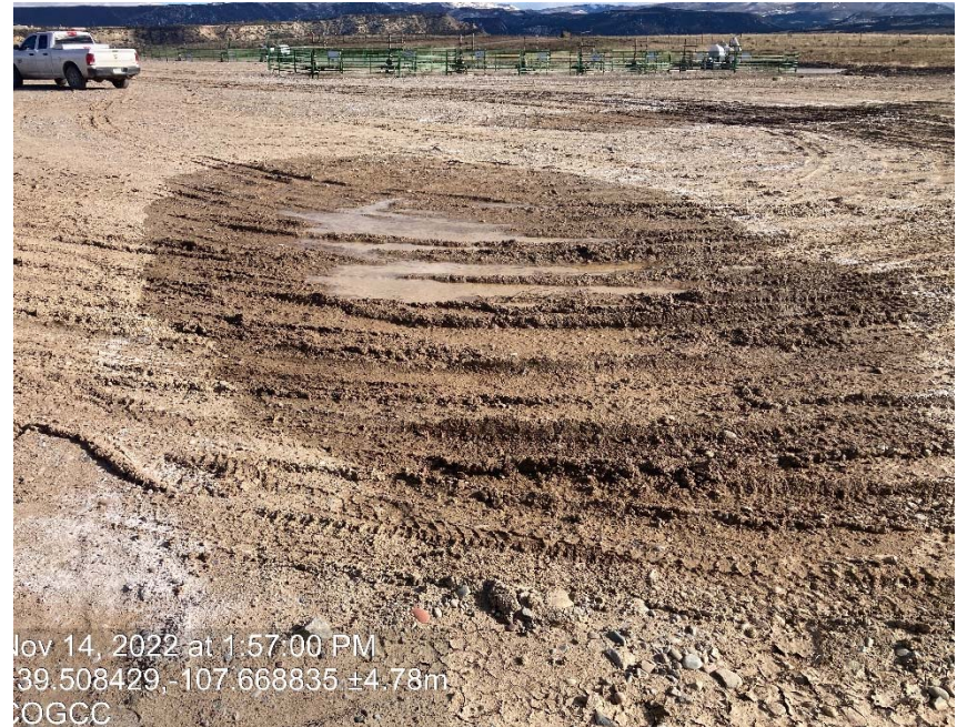
Lack of stabilization/ compaction
