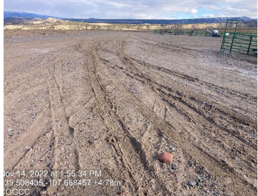
Lack of stabilization/ compaction
