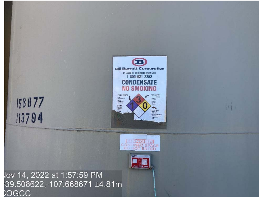
Tank label incorrect and lacking information
