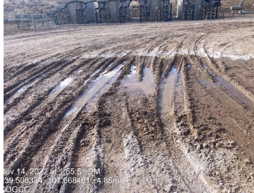
Lack of stabilization/ compaction
