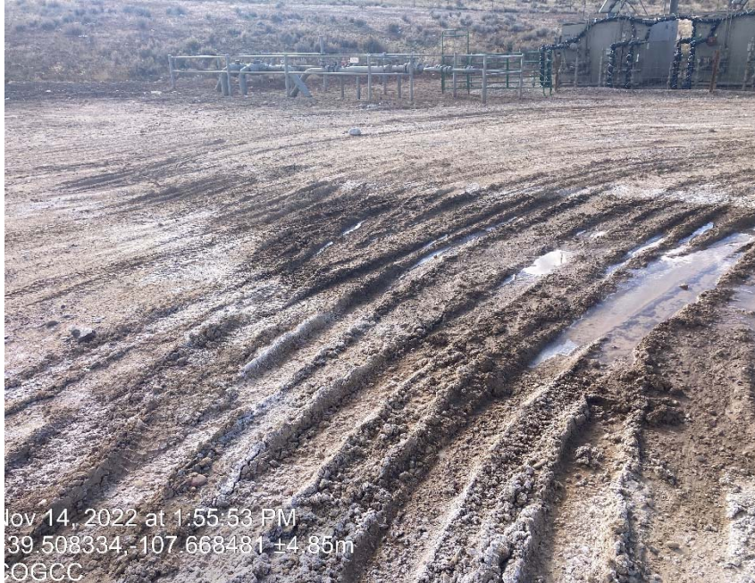
Lack of stabilization/ compaction
