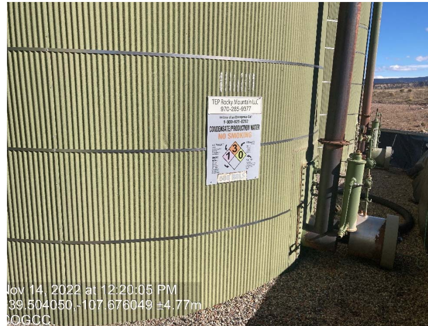
Tank label quantity faded
