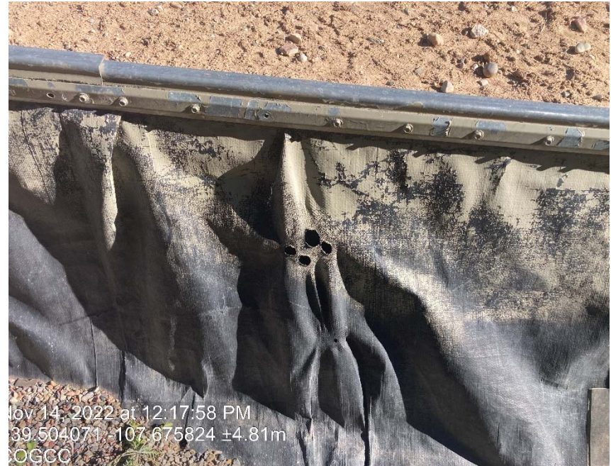
Holes in containment
