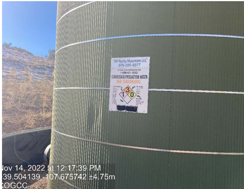
Tank labels missing quantity
