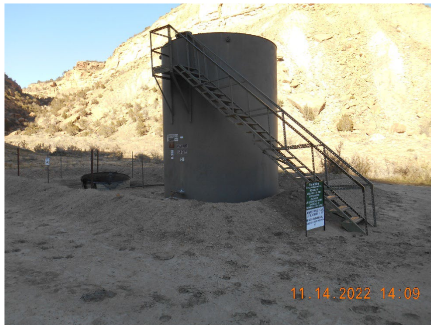
Condensate tank battery. Improper signs.
