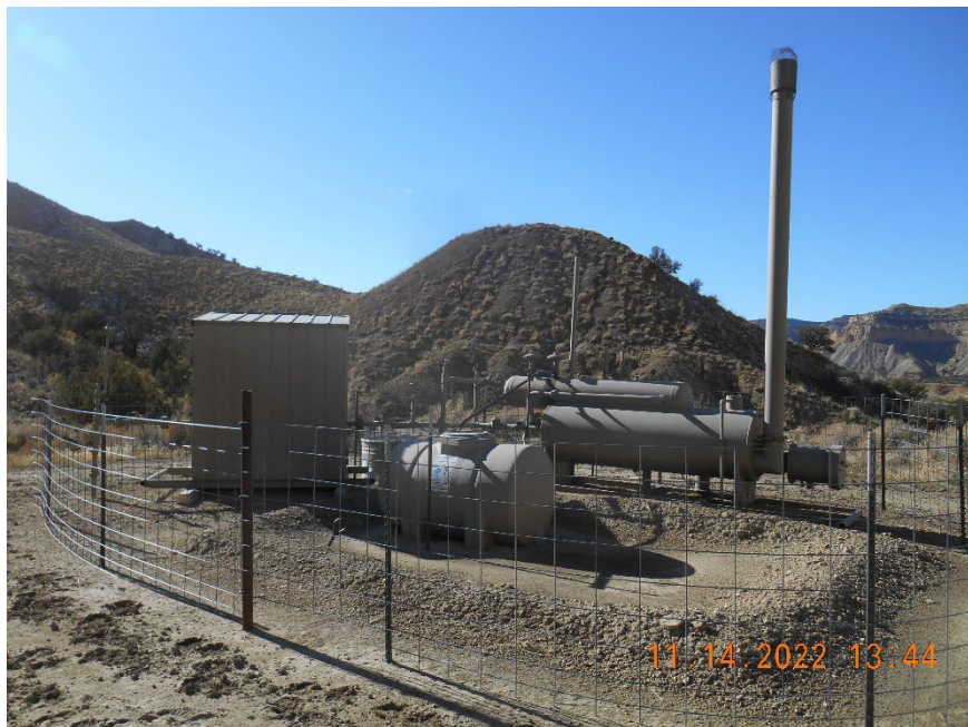
Meter housing, Separator with blowdown tank
