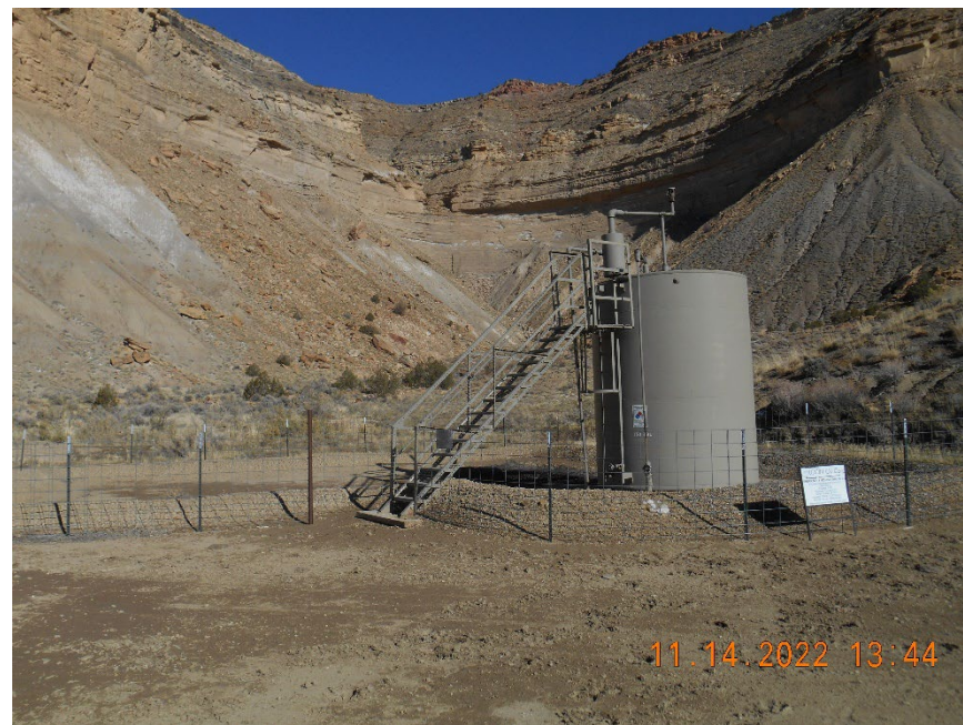
Condensate tank battery
