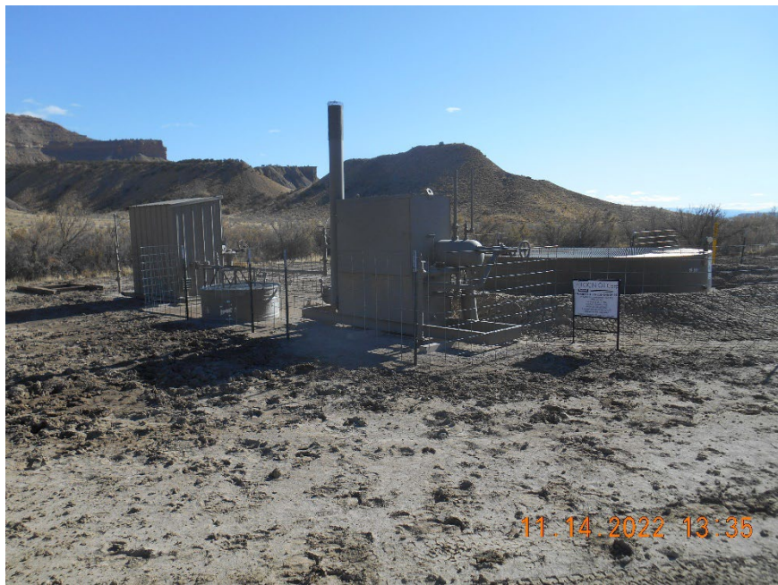
Meter housing, Separator with blowdown tank
