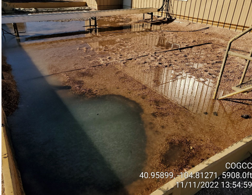
Photo 9 Standing liquid in containment at separator building
