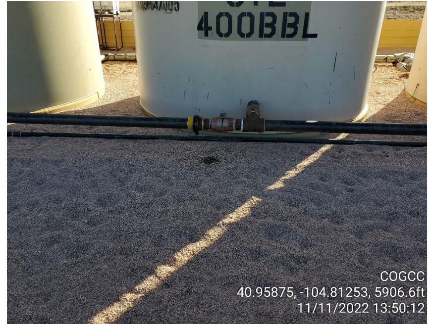
Photo 6 Leak at fittings on crude oil tank load line
