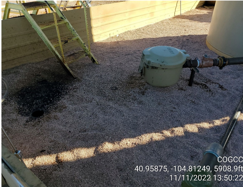
Photo 7 Staining around sump in northeast corner of tank battery
