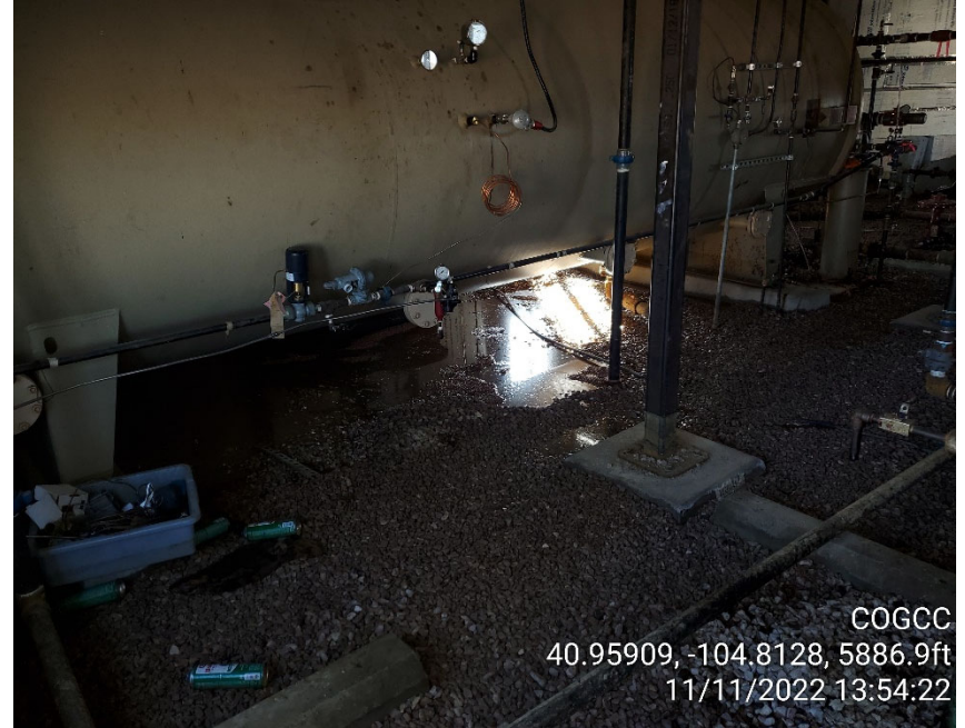
Photo 10 standing liquid inside separator building
