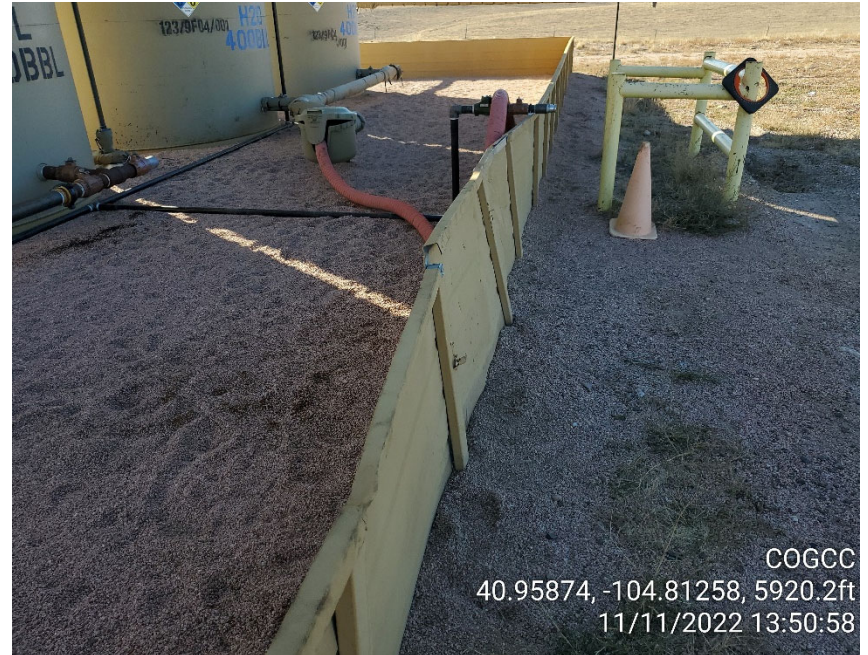
Photo 8 Damaged containment wall on north side of tank battery
