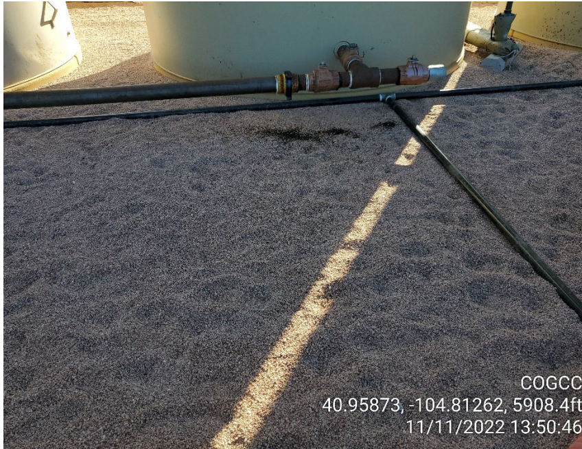
Photo 5 Leak at fittings on crude oil tank load line
