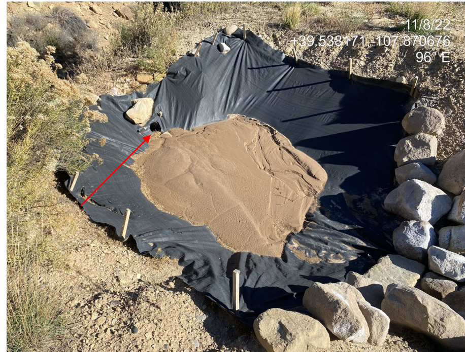
Photo 8. Photos show stormwater BMPs at the east of the Location. Sediment trap is not in proper functioning condition; sediment has reached the level of the drain resulting in reduced ability for trap to settle sediment.
