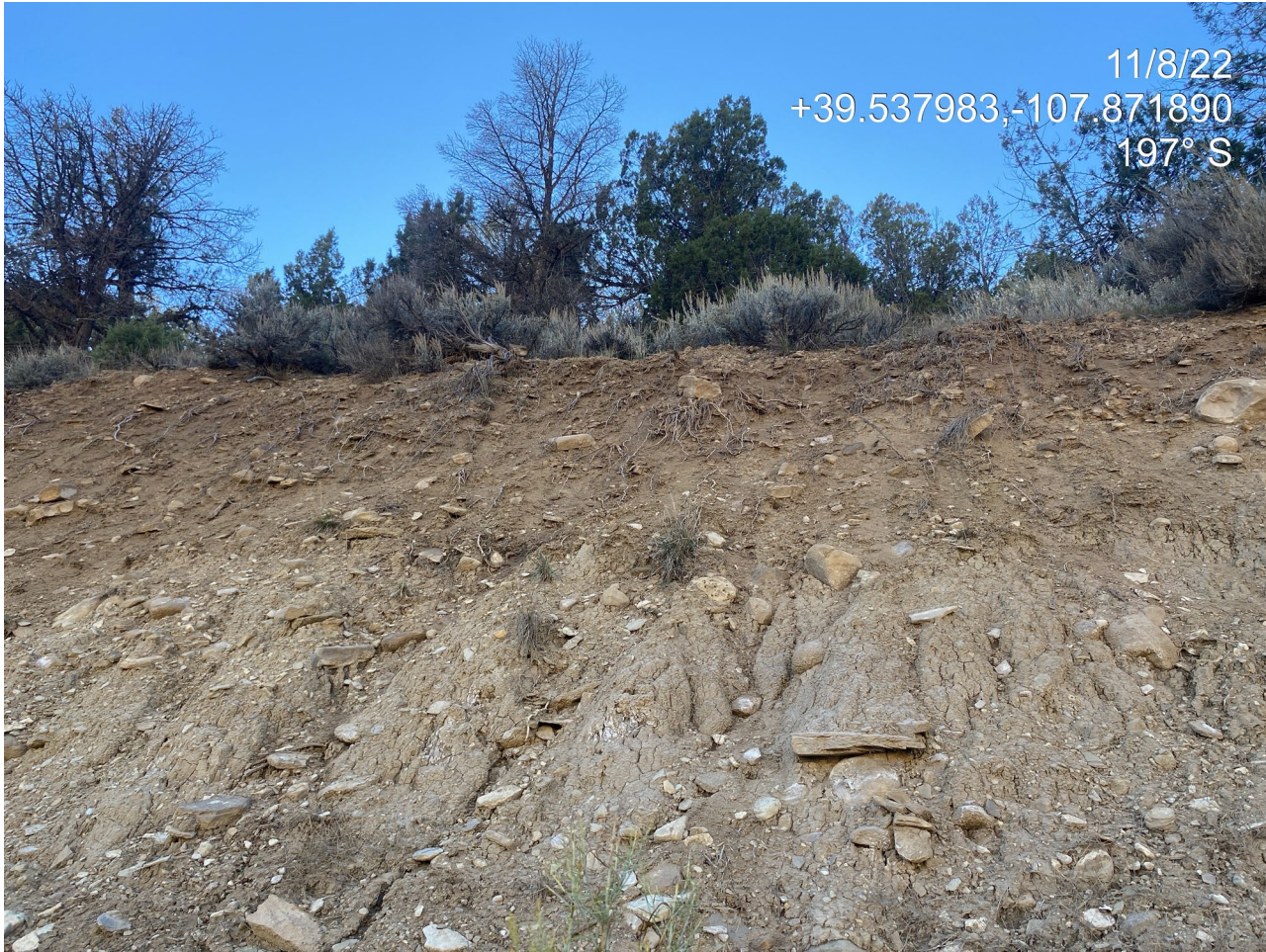
Photo 5. Photo shows exposed, undermined roots on the bare, eroded cut slope at the south of the Location.
