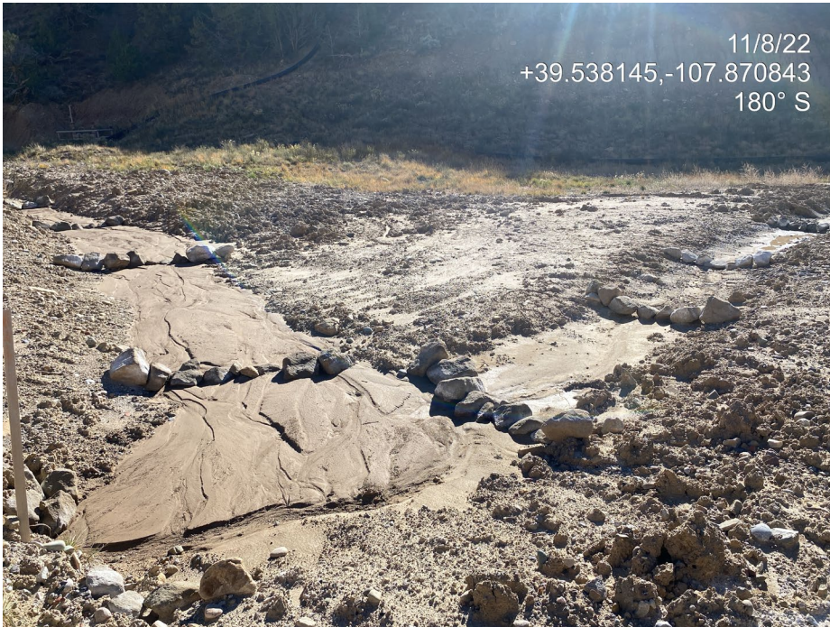
Photo 7. Photos show stormwater BMPs at the east of the Location. Bare exposed soils are prone to erosion and are resulting in high sediment loads.
