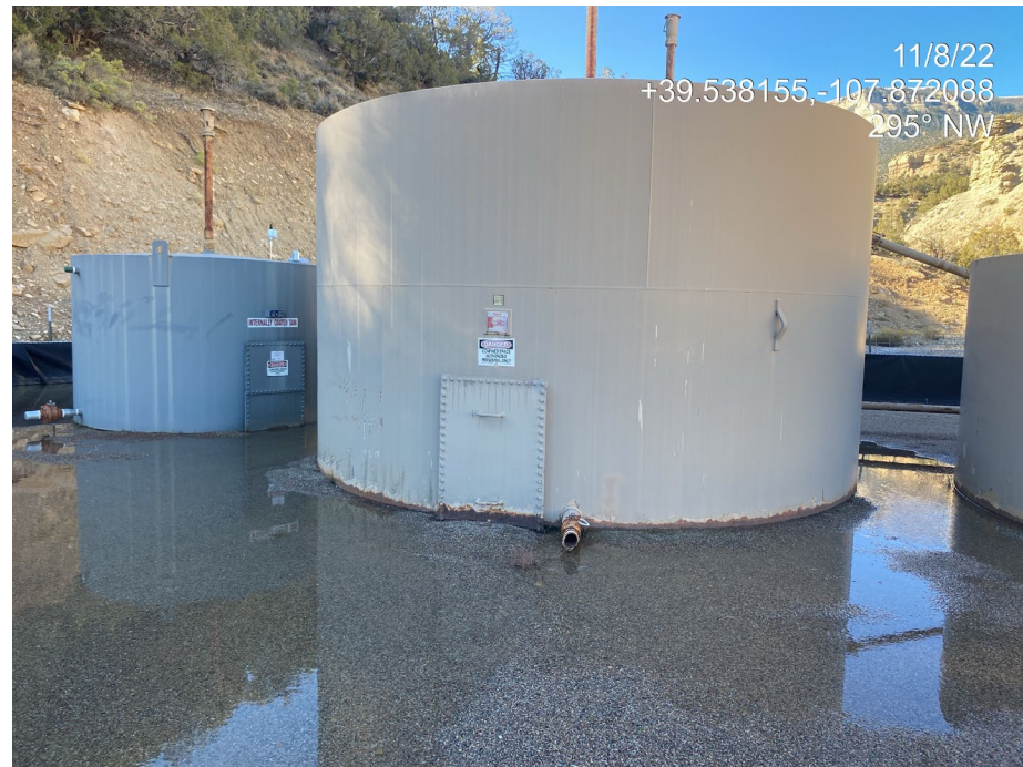
Photo 3. Photo shows tank drain line missing a bull plug.
