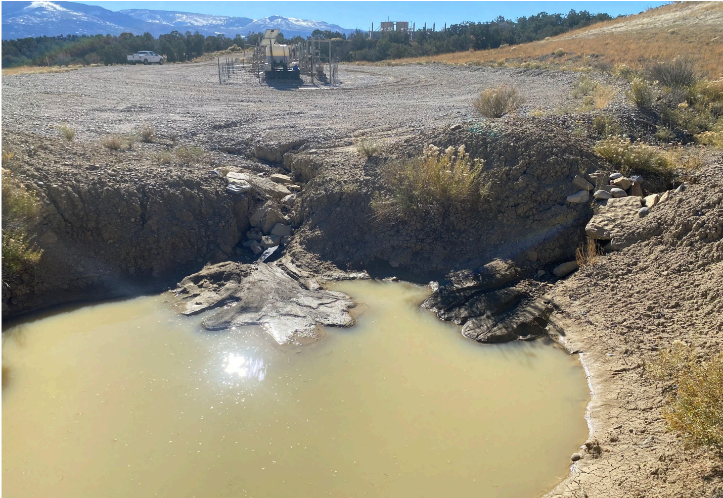
Photo 9. Photo shows an example of a sediment trap inlet where concentrated flows cutting are beneath rock armor. No geotextile liner was observed.
