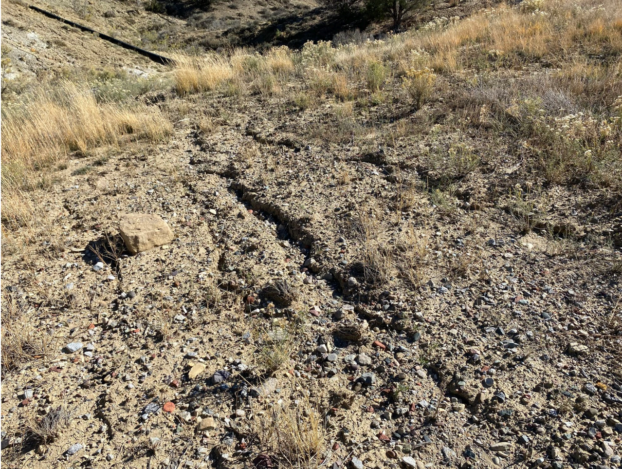
Photo 5. Photo shows rill erosion occurring in portions of the interim area/fill slope to the east. Current vegetative cover is insufficient to stabilize the slope.
