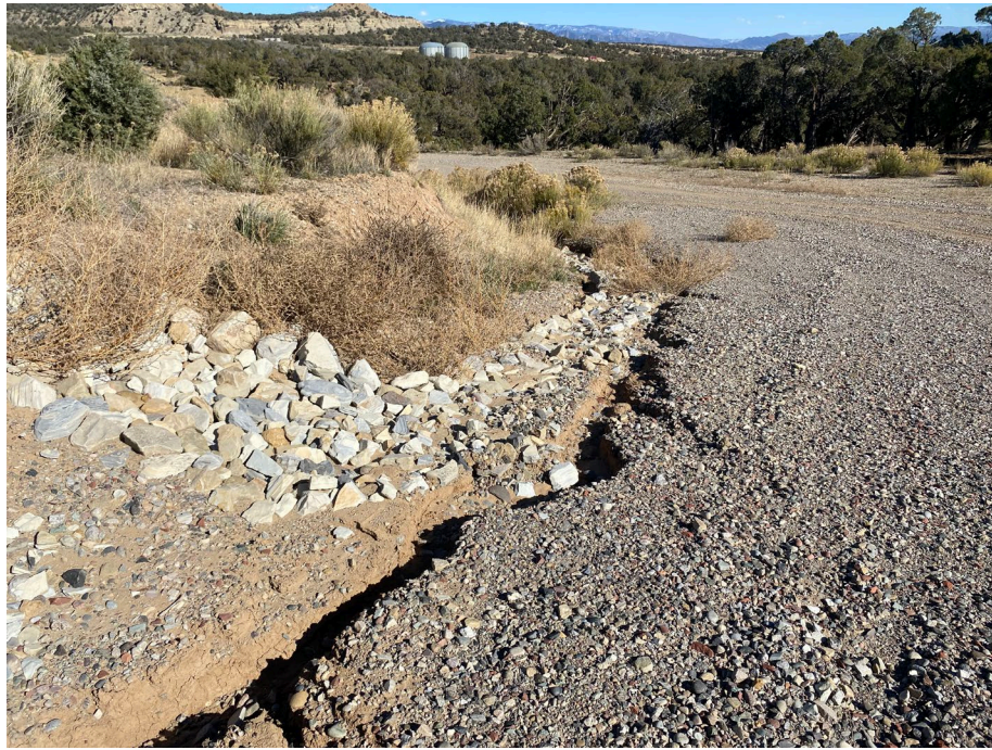
Photo 6. Photo shows erosion degradation migrating from the separators to the access road. Stormwater is cutting beneath rock armor, no geotextile liner observed.
