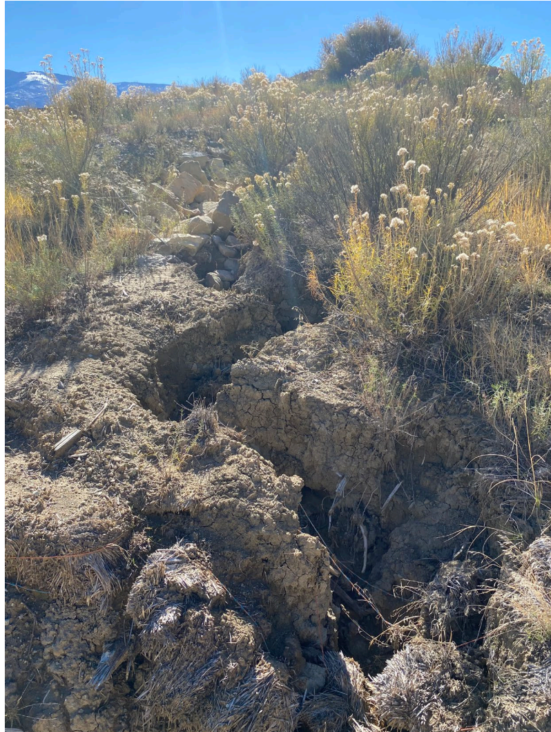
Photo 10. Photo shows an example of a erosion degradation occurring at a sediment trap outlet.
